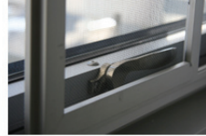
Above: Operable windows allow letting in outside air during temperate times.
