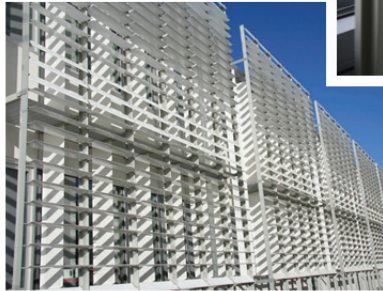
Below: Mechanical sun panels control the amount of natural light entering the building.
