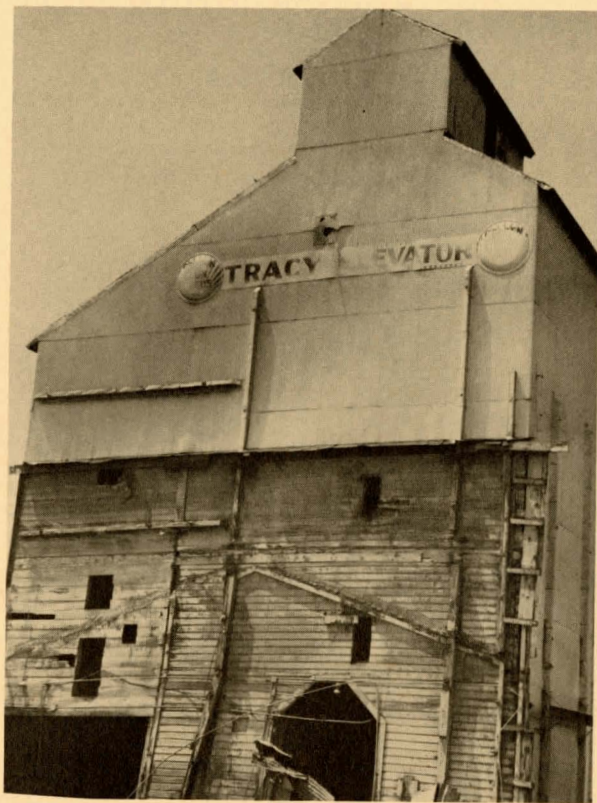
Grain Elevator. Tracy. Dismantling reveals the structure of the elevator.
