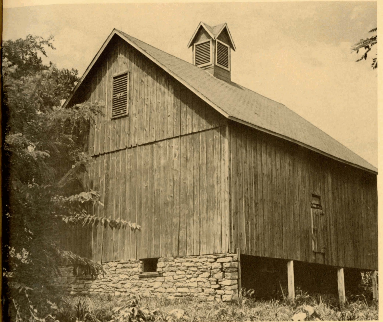
Barn. Knoxville. On the lower level, the German style barn has a sheltered entry for the livestock and on the opposite side a ramp for entering the upper level.
