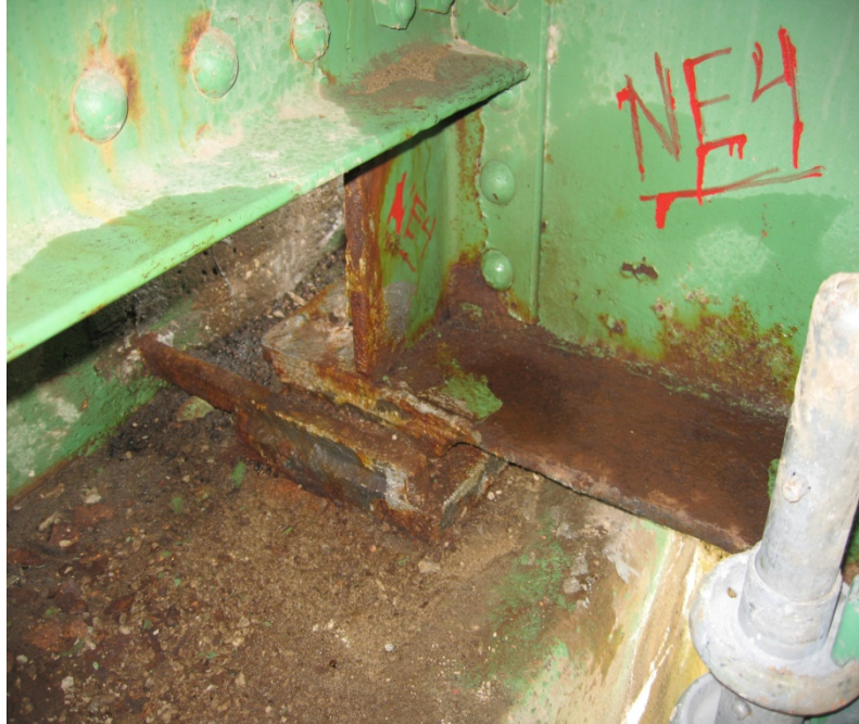
Figure 4.46 Forced vibration response measurement of northeast end and boundary condition of beam 4 with noticeable deterioration of the bottom flange
