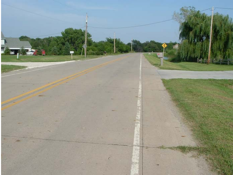
Figure 4. Paved shoulder with maintainable slopes
