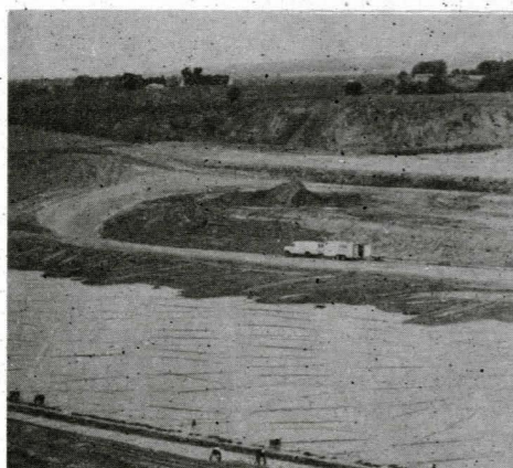
On August 23, 1995, the Harrison County Landfill opened its doors and began receiving solid waste from county residents. The composite liner used in the landfill consisted of two feet of compacted sub-base and a 60 mil HPDE plastic liner.
