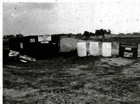
During the construction of Metro Waste Authority's Regional Collection Center in Bondurant, C&D waste was collected and separated. The waste was then sent to a recycler for processing.
