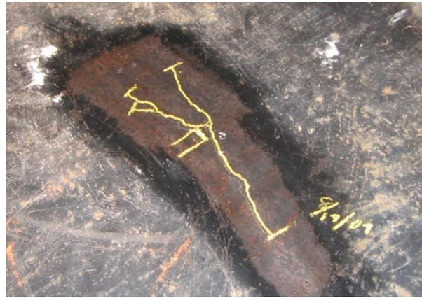
b. Close-up of top web plate cracking
