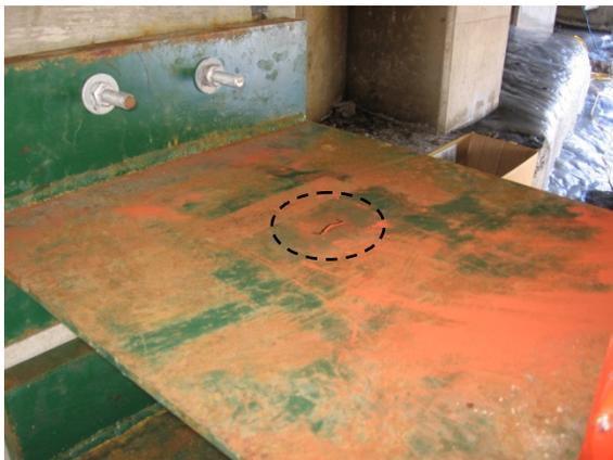
b. Top Web-Plate Cracking
