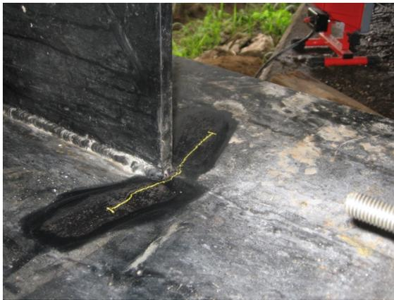
c. Bottom web plate cracking
