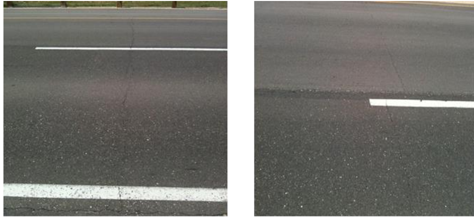
Figure 44. Longitudinal joint performance for the IA 13 project
