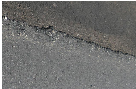
Figure 2. Butt joint construction with hot pinch (pictured on US 61)
