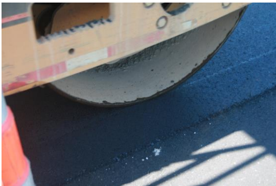
Figure 2. Butt joint construction with hot pinch (pictured on US 61)
