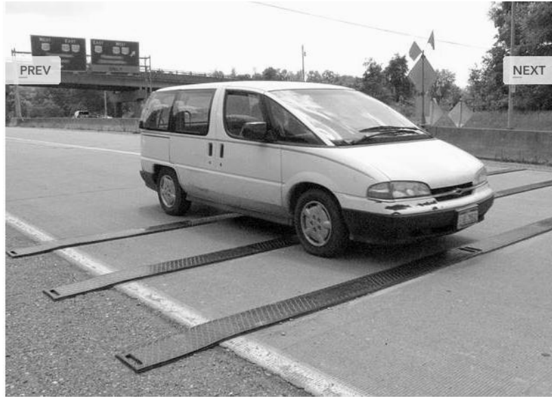
Figure C.1. Temporary rumble strips
