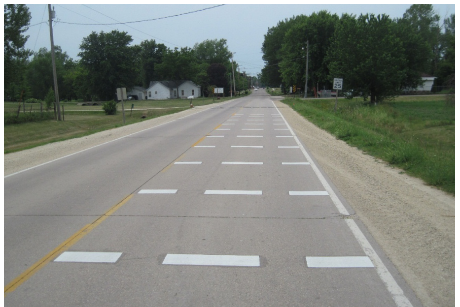
Transverse bar treatment at Hazleton east entrance
