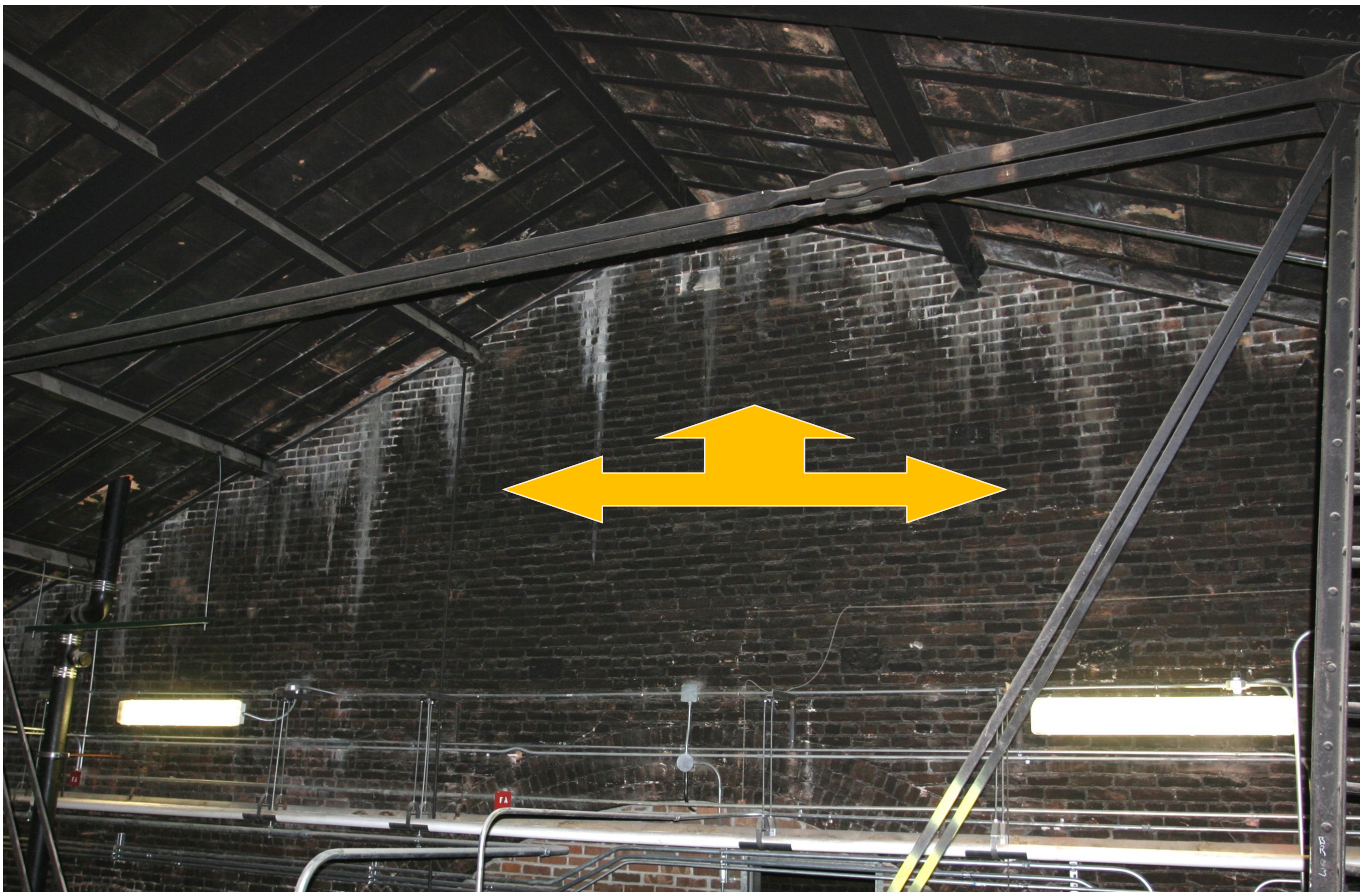
Soot covers the north wall and ceiling of the attic above the House Chamber. Water used to fight the fire streaked areas of the brick wall.
