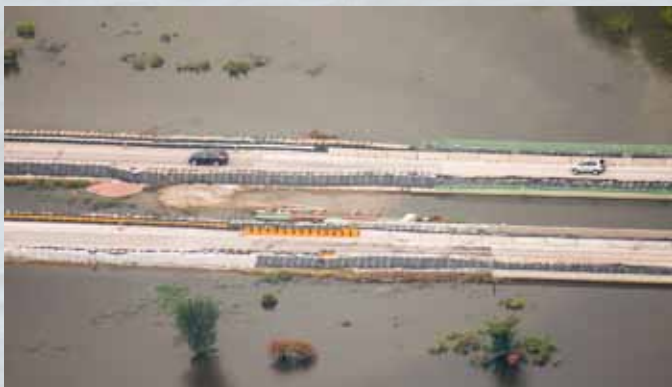
Using the LiDAR technology, Iowa DOT engineers were able to precisely pinpoint locations on Interstate 29 in jeopardy of being overtopped by the Missouri River flooding. The flood risk at those locations could then be mitigated with equipment like the TrapBags seen here.
