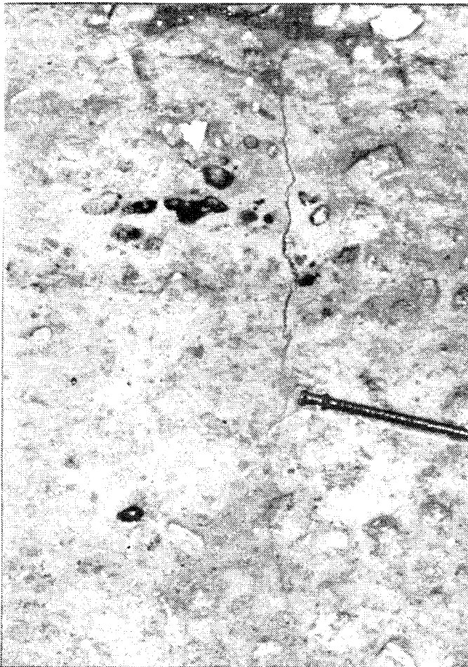
Photo 5 - A longitudinal crack in the substructure of pier MS-2
