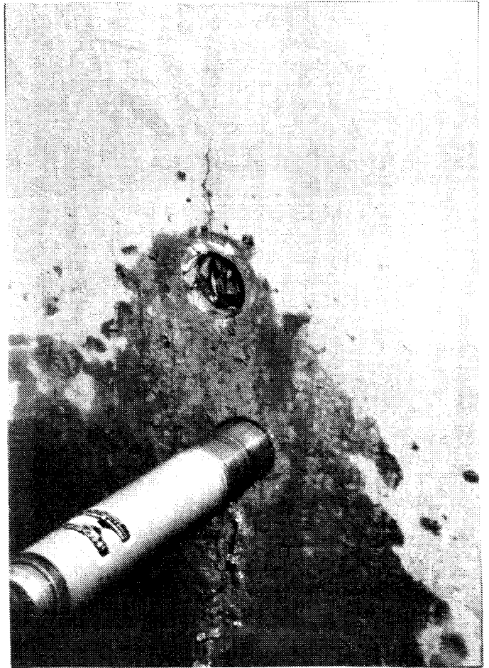
Photo 6 - Drilling cores in pier MS-2
