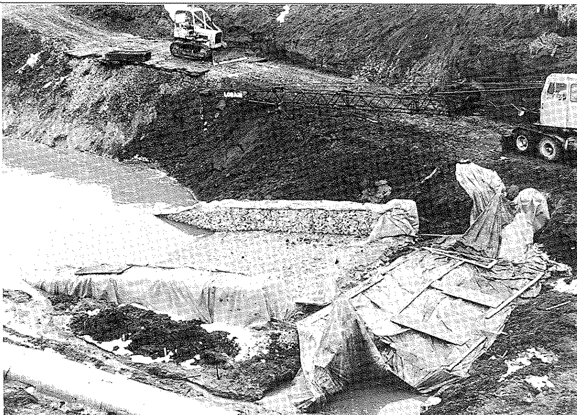
Plate A-2. Gabion spillway in place, Feb. 10, 1983.
