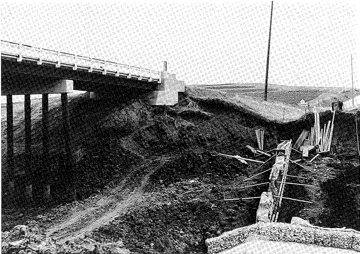
Plate A-5. Concrete cutoff wall at crest of structure, Apr. 27, 1983.
