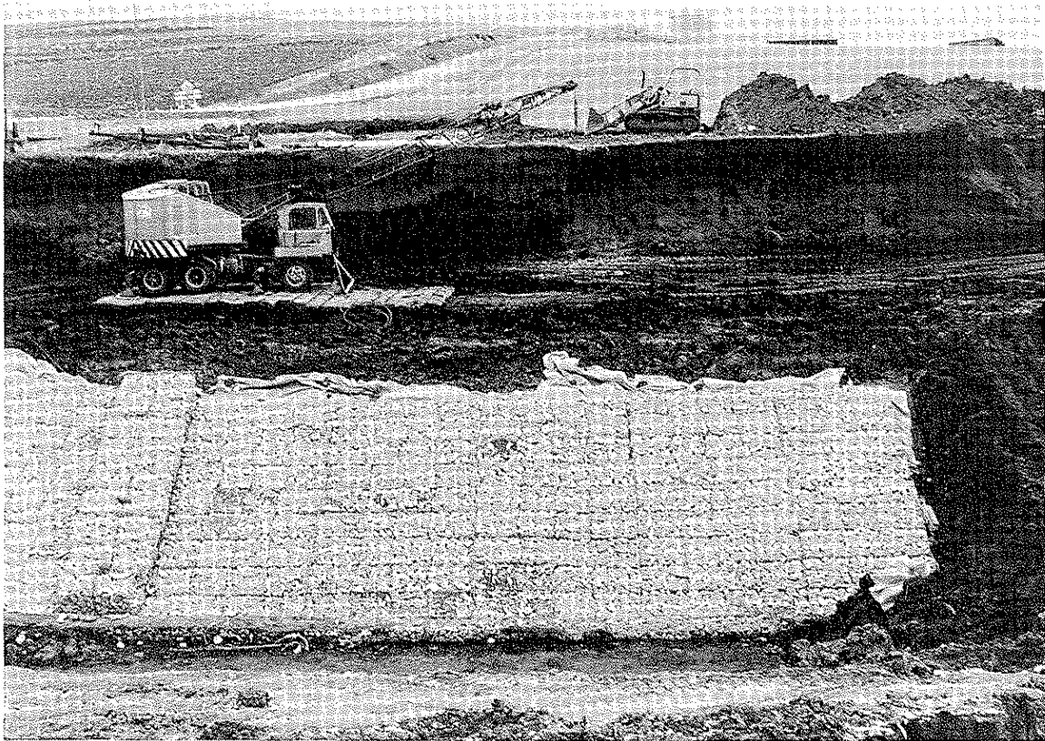
Plate A-4. Gabions in place on east side of spillway, Apr. 27, 1983.
