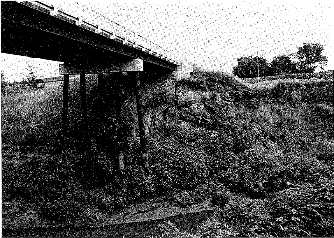
Plate 4. East end of bridge showing exposed piling and soil slide away from abutment. Light colored portion of the bottom of piles indicates where soil formerly covered piles, July 1979.
