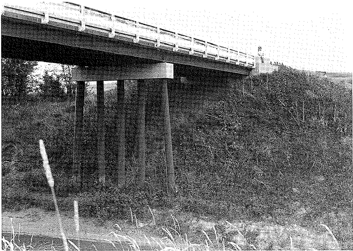
Plate 5. East end of bridge showing piling once again covered by soil and stable soil slope beneath abutment, June 1985.
