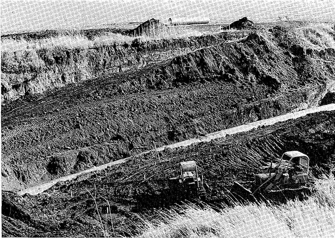
Plate A-1. Excavation and grading of side slopes, Dec. 18, 1982.
