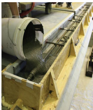
a) Pouring of UHPC at one end of the longitudinal joint
