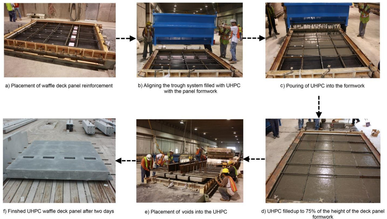
Figure 2.9. Construction sequence used for the UHPC waffle deck panels at the precast plant
