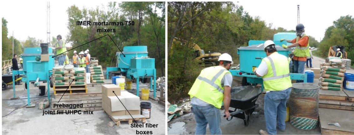
Figure 3.8. Batching of UHPC joint fill using IMER Mortarman 750 mixers at the bridge site
