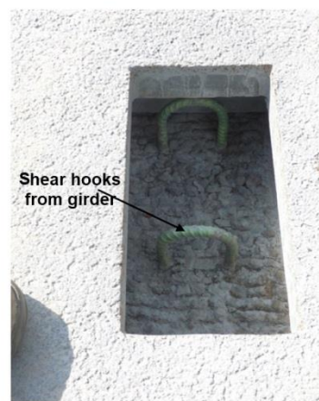
d) Shear pocket ( panel-to-girder connection)
