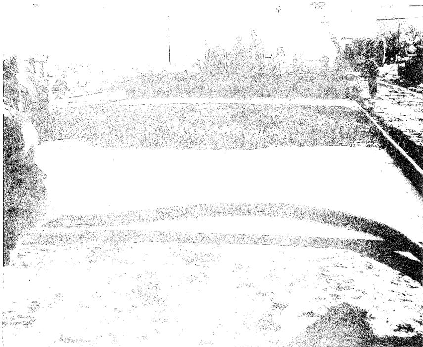
Photo 5: Concrete being placed on the Styrofoam.
