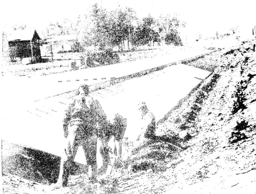
Photo 7: Styrofoam being placed on the 2:1 Slope in the Shoulder.
