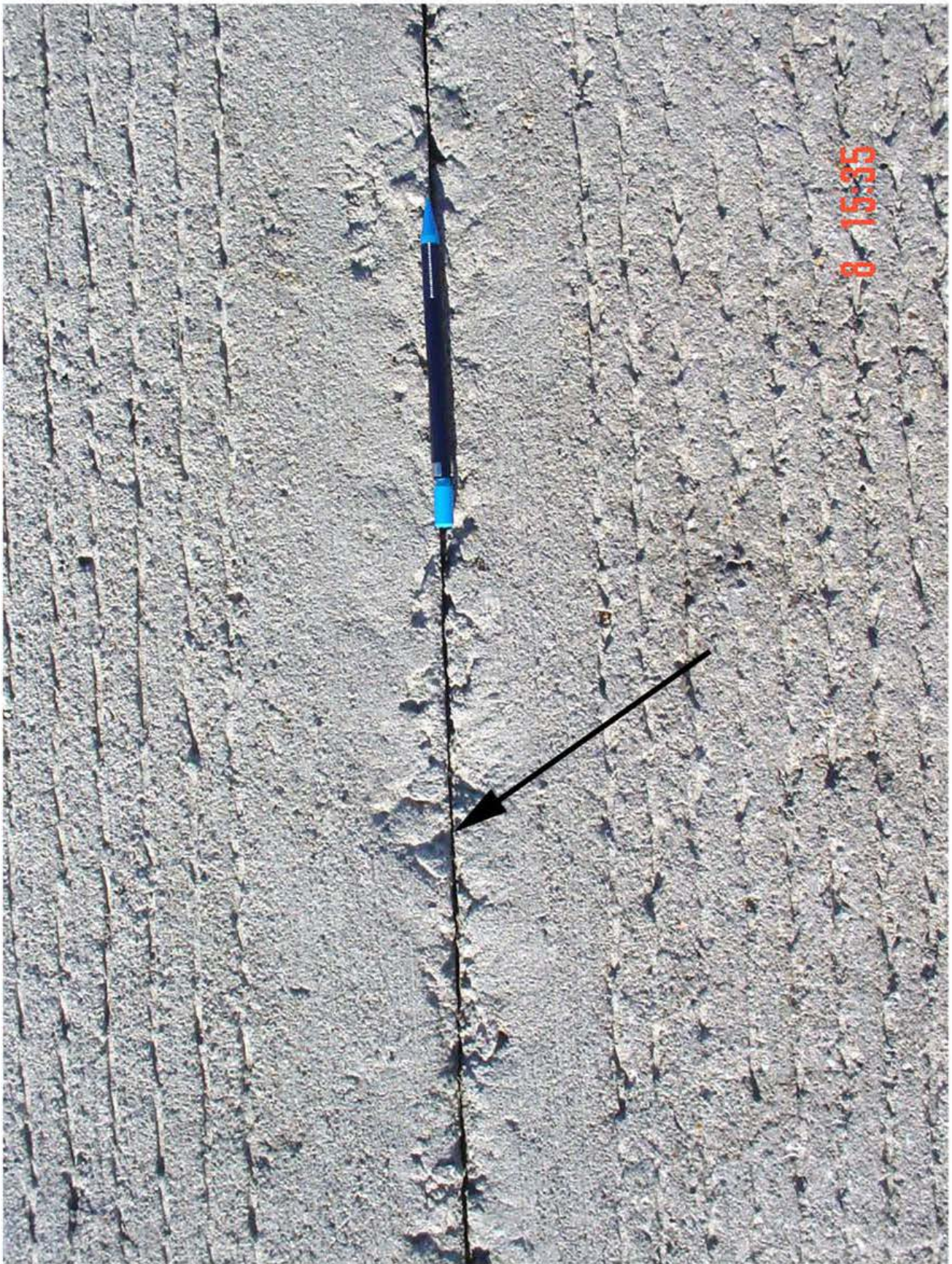
01) Hwy 218, NBL, Sta 838+50, Mt. Pleasant, Henry Co. 1/8/03 Open formed joint left by wide knife.
