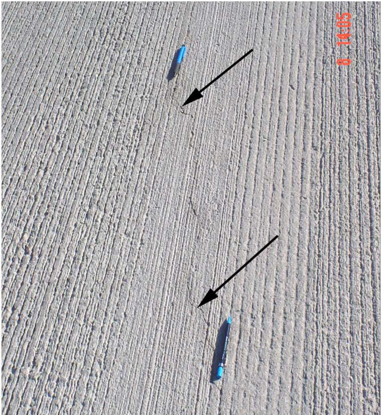
07) Hwy 92, CL Sta 280+06, Washington, Washington Co. 1/8/03 Random crack, 8' long, at beginning of joint test section.
