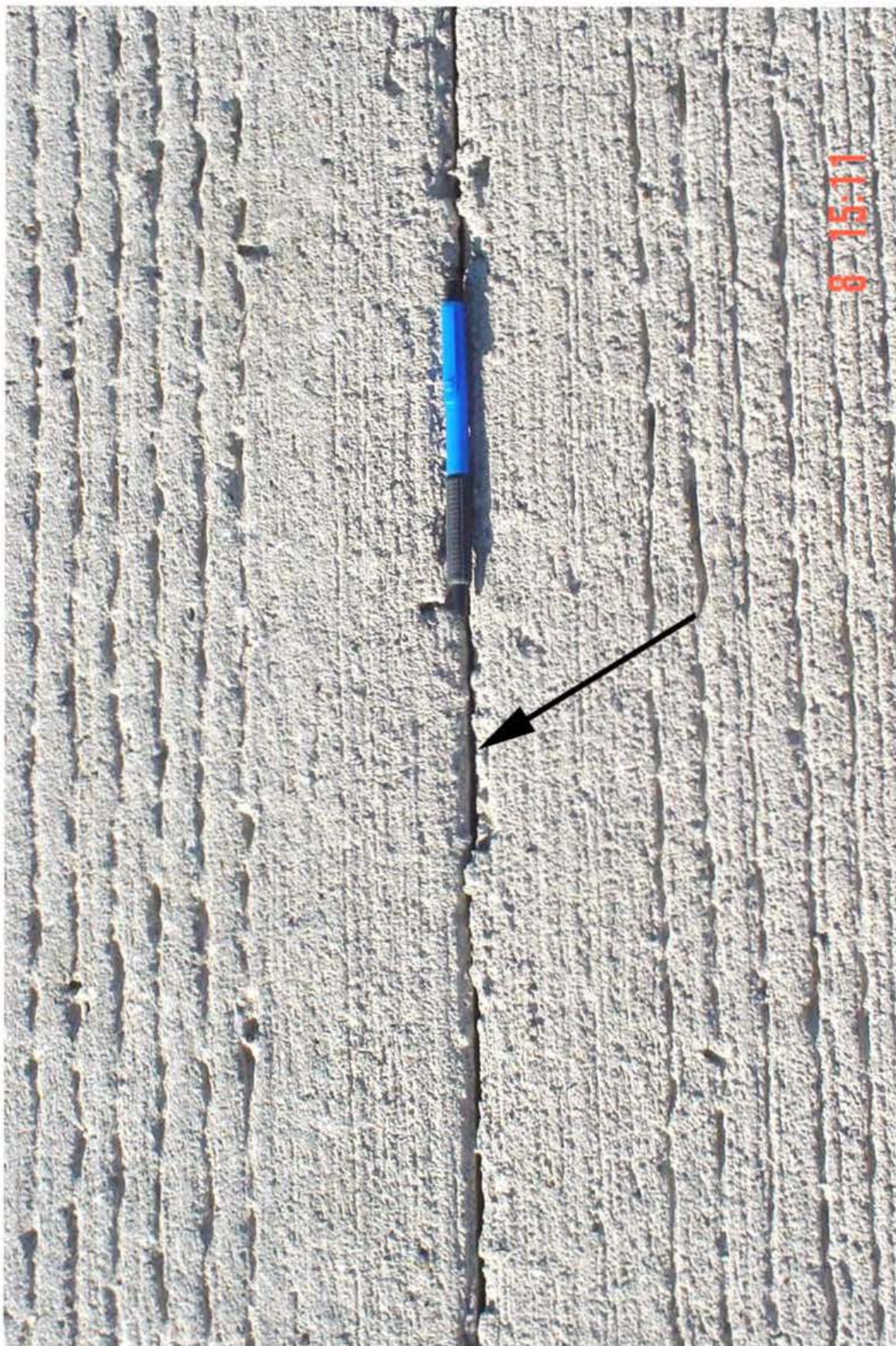
02) Hwy 218, SBL, Sta 863+37, Mt. Pleasant, Henry Co. 1/8/03 Open formed joint left by wide knife.
