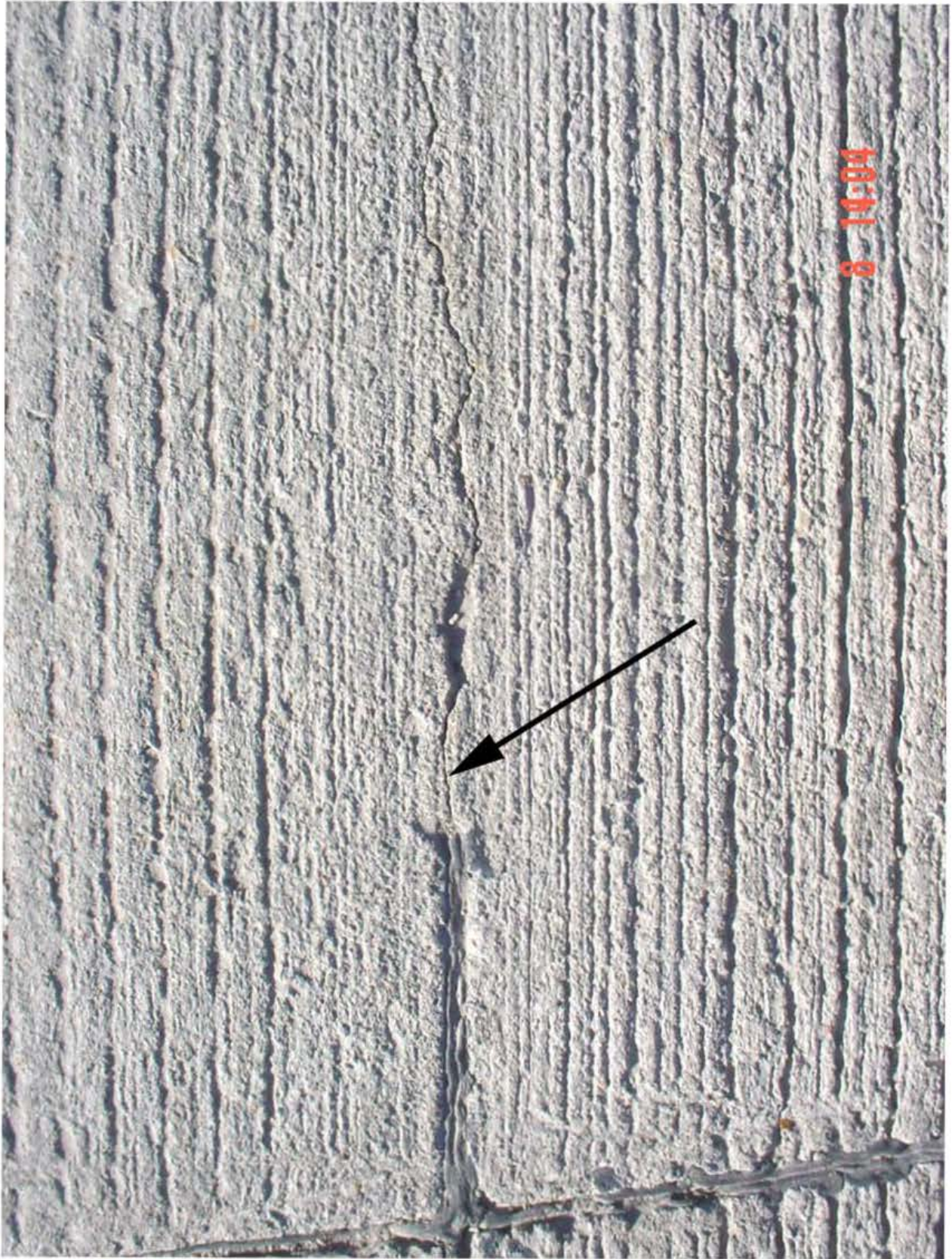
07) Hwy 92, CL, Sta 280+24, Washington, Washington Co. 1/8/03 Beginning of formed joint test section.
