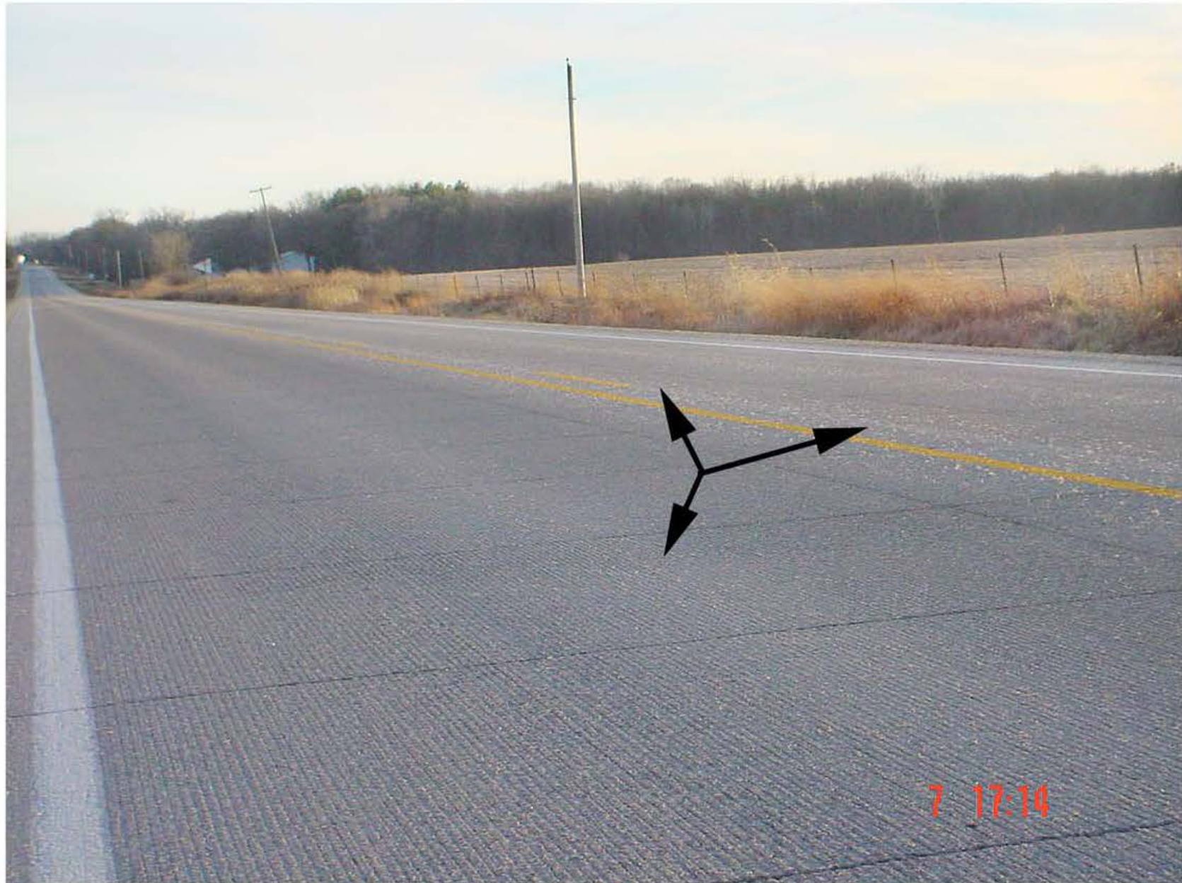
08) Hwy 13, Sta 85+00, Manchester, Delaware Co. 1/7/03 Formed joints 5 feet from each shoulder. Note white tips of fibers in the PCC.
