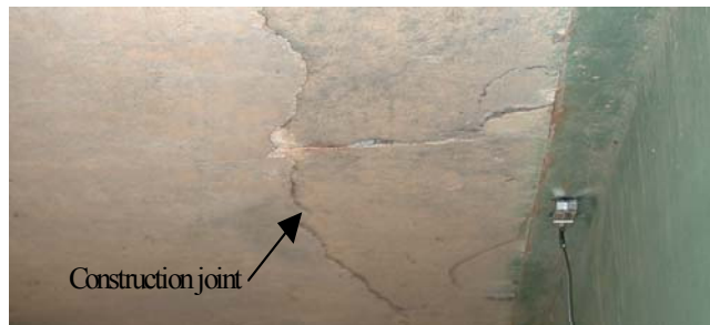
e. Concrete cracks.
