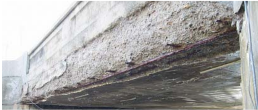
a. Spalling and heavy deterioration at edge.
