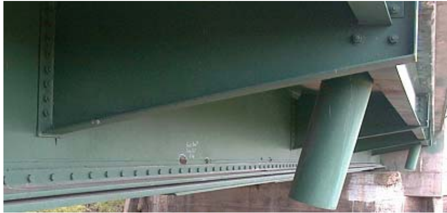
c. The non-uniform section bolted to the main girder.
