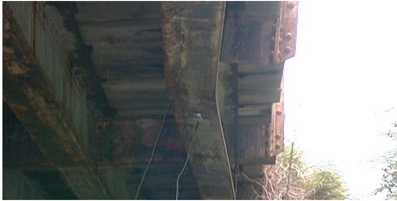
a. Bent girder on far West side at midspan.
