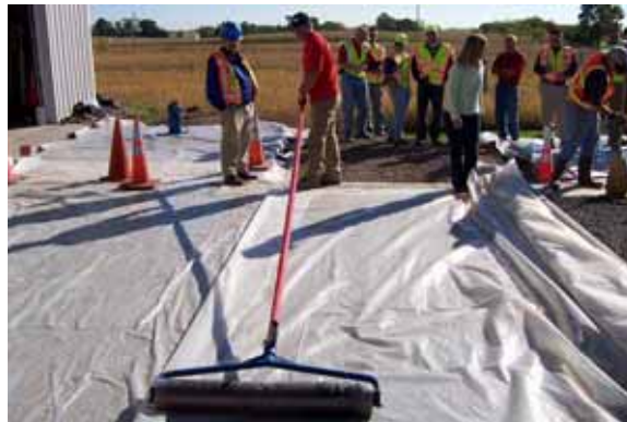
Figure 4. Transverse steel roller over the moisture barrier
