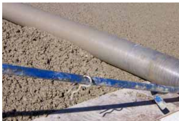
Figure 5. Compaction and finishing using a roller screed
