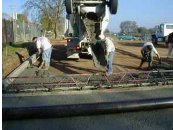
Figure 3. Vibratory screed used in placing PCPC
