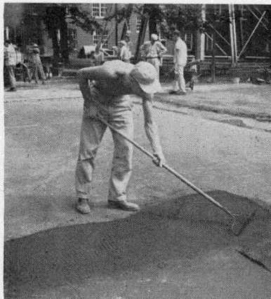
Fig. 35. Laying a test pavement by hand.
