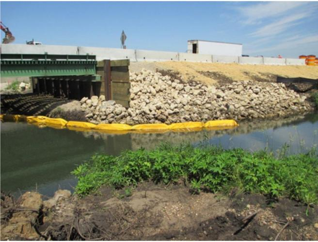
Figure 13 – BuchUp near bridge construction
