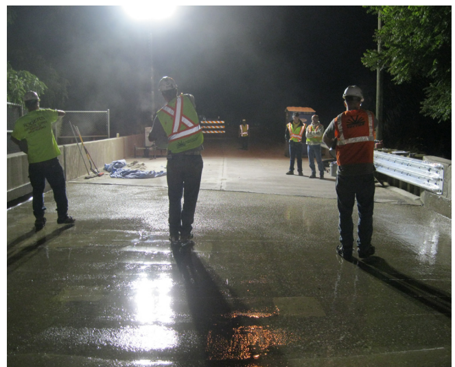
Hand-broadcasting flint chips on the first polymer layer of the Johnson County bridge deck
