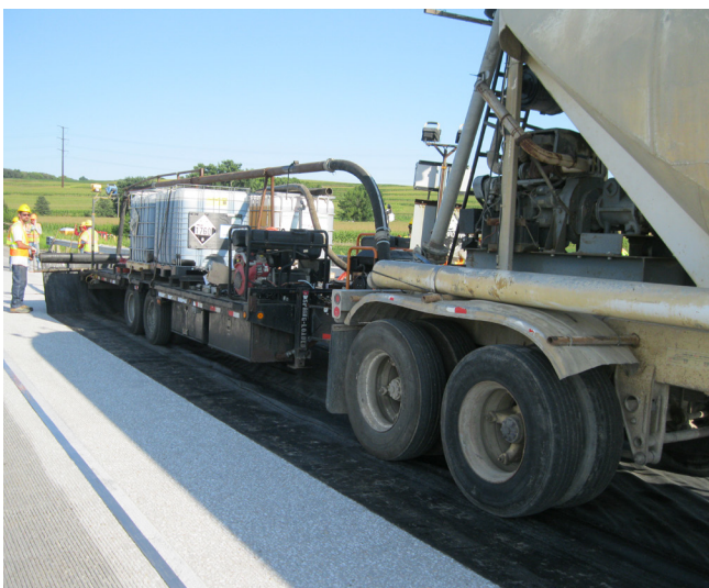
Semi-truck and trailer carrying hopper of flint chips, vats of epoxy polymer, and a blower on the Keg Creek Bridge
