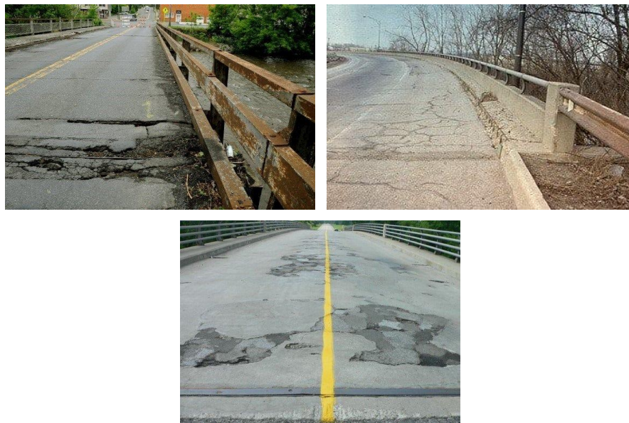
Figure 1.1. Typical examples of bridge deck deterioration
