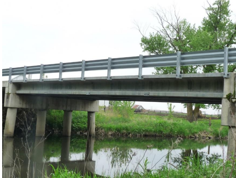
Figure 1.3. Jakway Park Bridge with UHPC pi-girders in Buchanan County, Iowa
