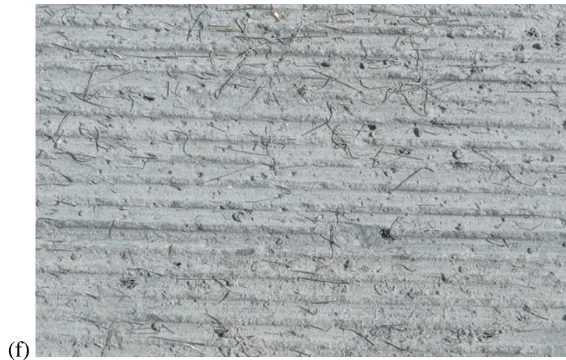
Figure 3.3. Overlay construction: (a) roughened deck surface prior to placing the overlay, (b) placing of the UHPC overlay with a screed, (c) UHPC overlay after casting one lane, (d) grinding of the surface, (e) grooving of the surface, and (f) close-up view of the finished surface
