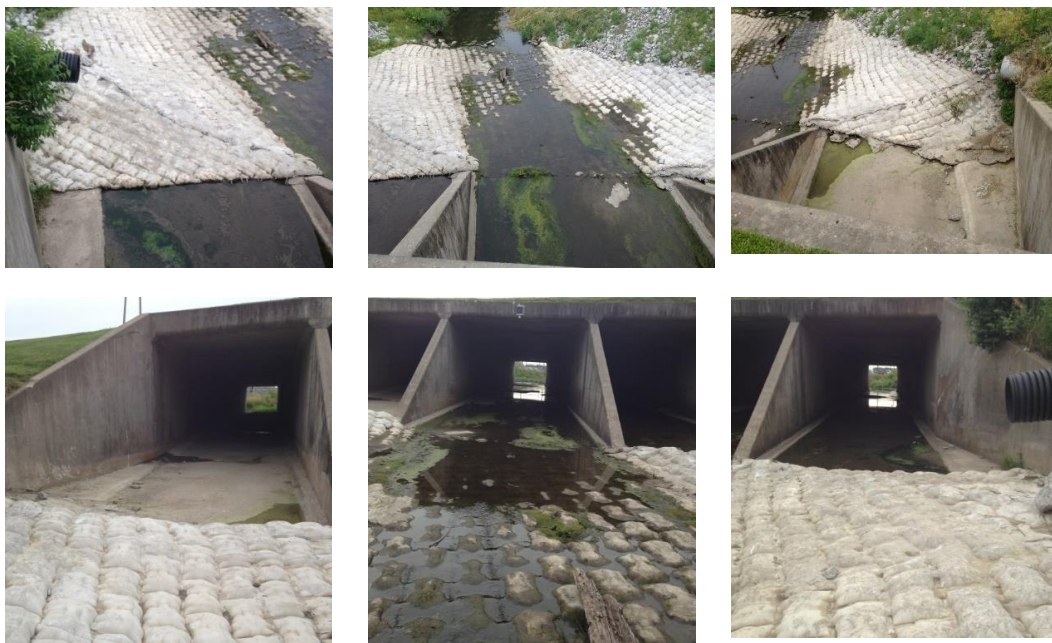
Figure 5A. Views of the mat-covered fillets as applied at the inlet of a 15'-18"-15" x 12 RCB on Hwy 1 W, Iowa City. Note: there is a slight difference in the fillet geometry compared to the specifications provided in Appendix A. The geometry has been updated based on observations during the monitoring of the implemented design.
