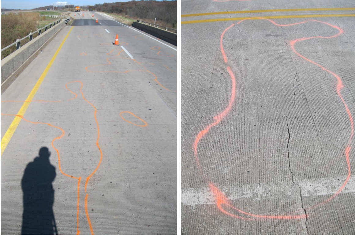
Figure 3.4. Photographic documentation of delamination
