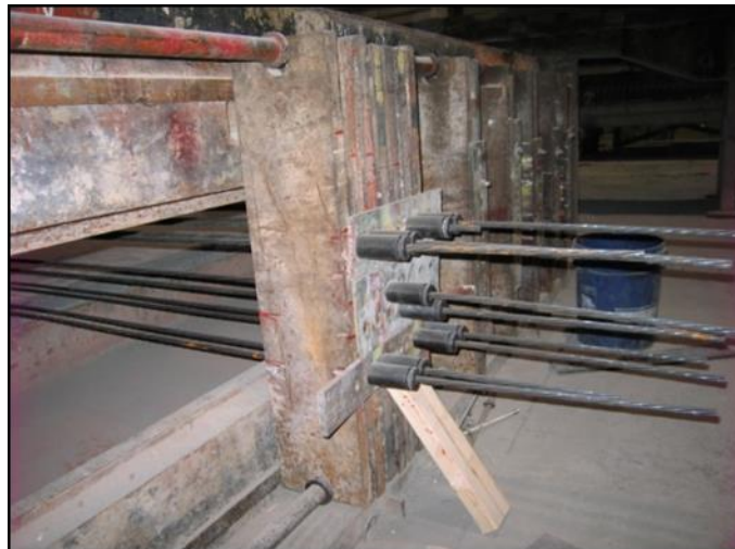
Figure 5-8. Prestressing strands layout at the anchorage end
