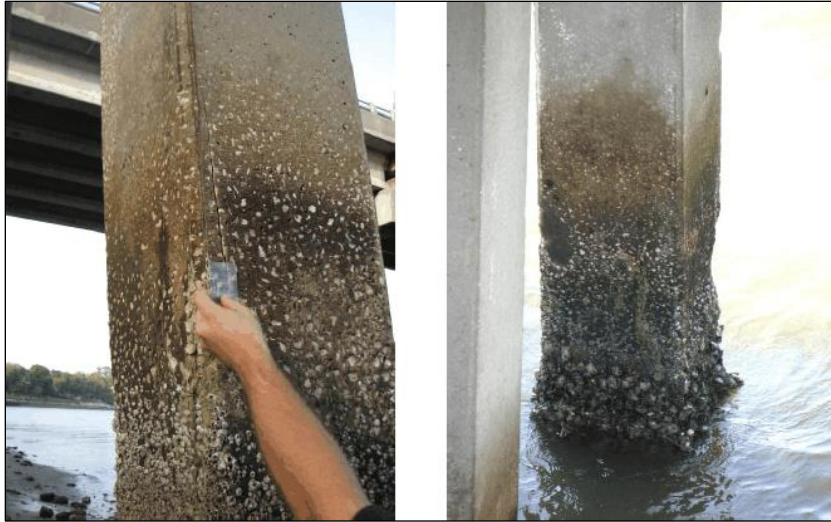
Figure 1-3. Damage to prestressed concrete pile due to corrosion
