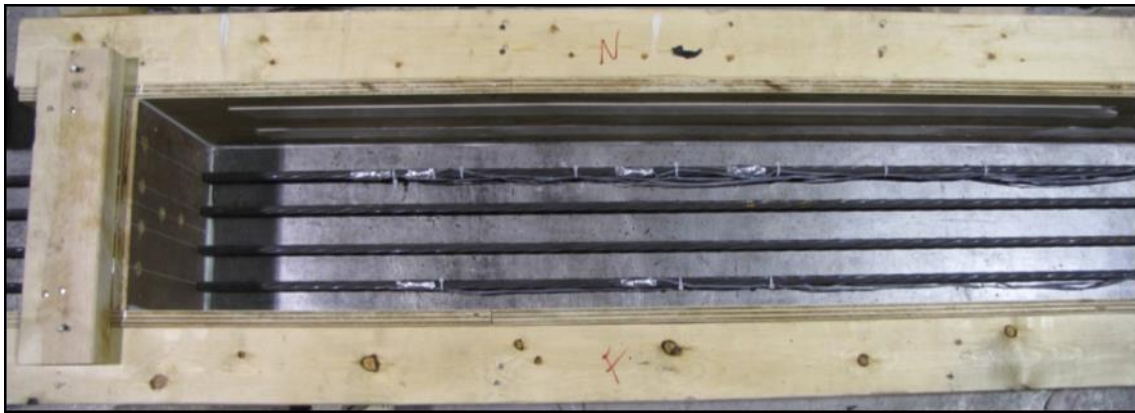
Figure 5-7. Instrumented bottom prestressing strands in the form
