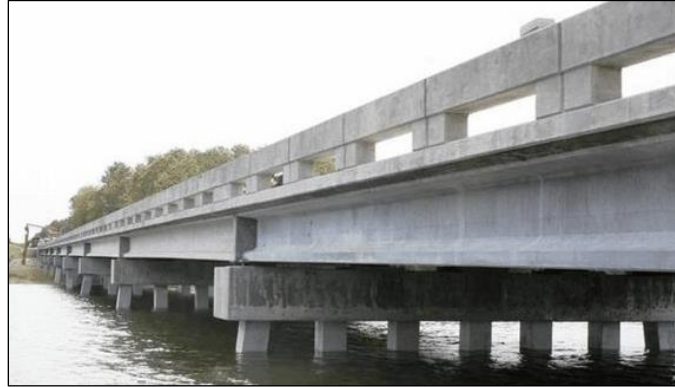
Figure 2-6. Cat Point Creek Bridge with UHPC girders on one span in Virginia
