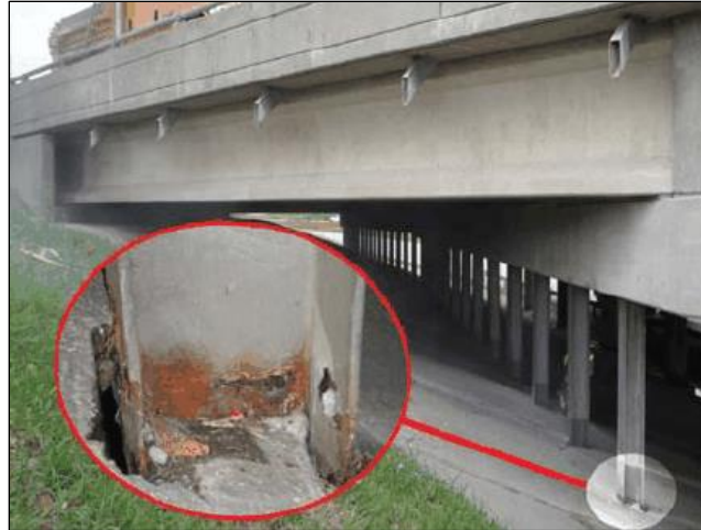
Figure 1-6. Corroded steel H-pile
