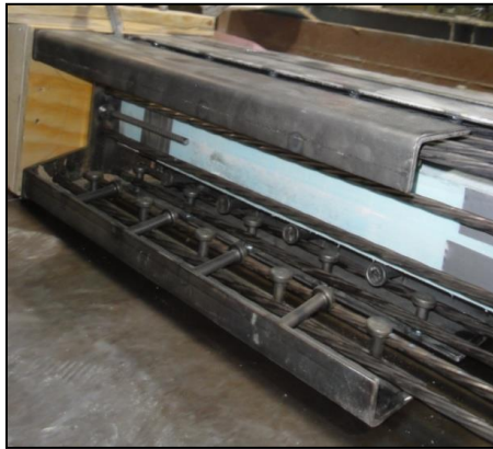
Figure 6-11. Splice at a UHPC pile end prior to placing the formwork
