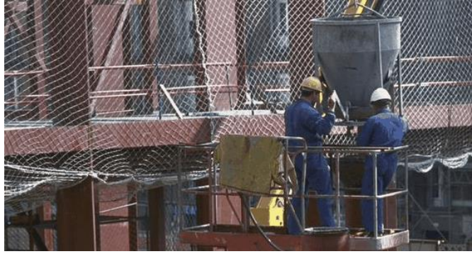
Figure 2-8. Onsite pour for UHPC columns during Queen Sofia Museum expansion
