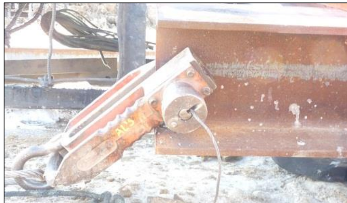
Figure 7-17. Steel HP 10 × 57 production pile pickup point
