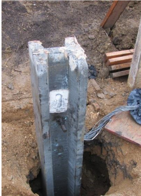
Figure 7-20. UW1-2 after installed in the prebored hole
