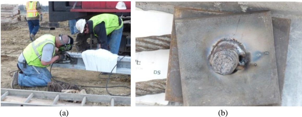
Figure 7-15. (a) Welding the 2nd washer to the threaded rod and (b) pickup point after welding
