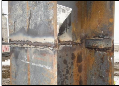
Figure 6-24. Steel HP 12 × 53 butt-weld splice
