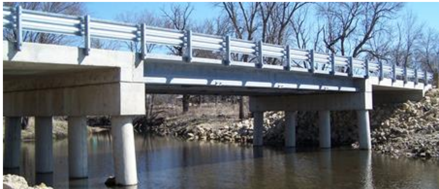
Figure 2-7. Jakway Park Bridge in Iowa using Pi-girders
