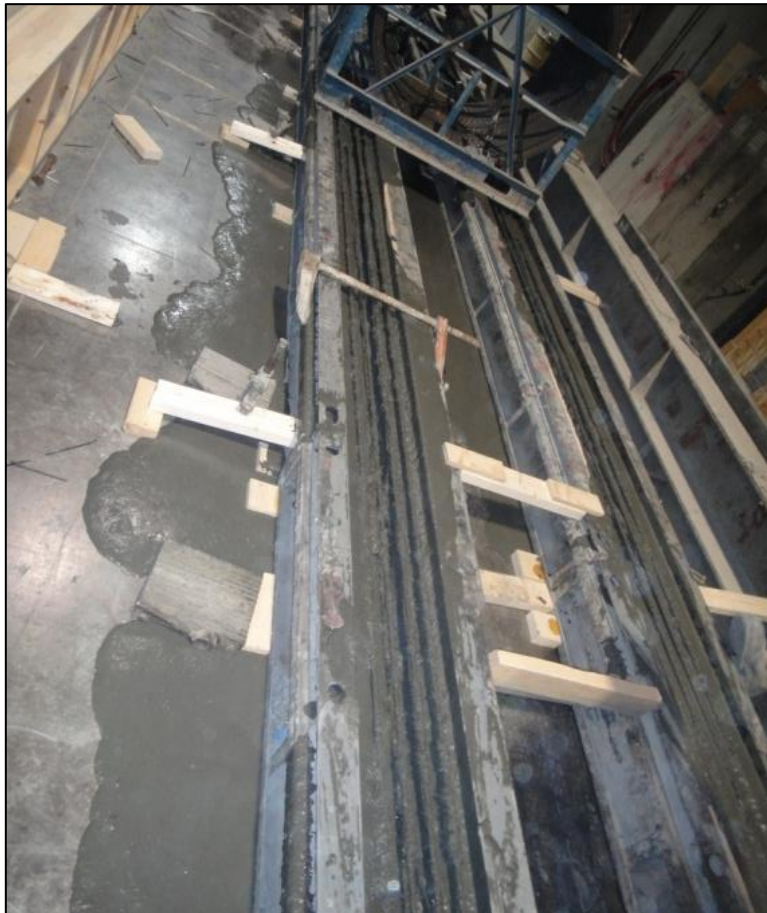
Figure 6-16. Steel forms beginning to tilt causing UHPC to leak
