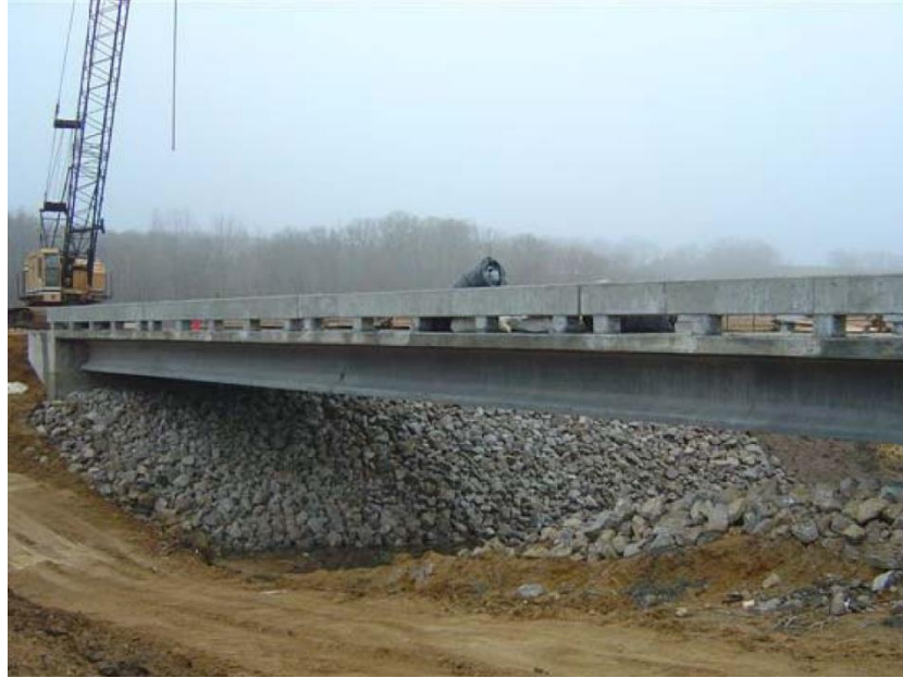
Figure 2-4. The UHPC girder bridge in Wapello County, Iowa
