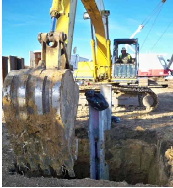
Figure 6-53. Excavation of soil surrounding P4
