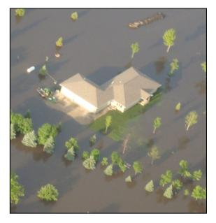
Figure 11-2 A new building elevated on fill plus freeboard was not damaged by this flood
