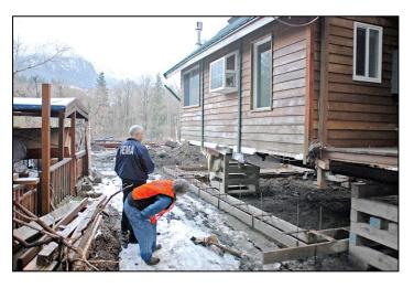
Figure 12-17 In-process elevation project to bring a substantially damaged building into compliance
