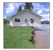
Figure 1-6 Riverine erosion can undercut structures
