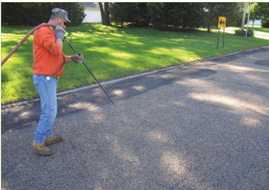
Figure 3–45. Cleaning the existing pavement surface (CCEE/ISU)
