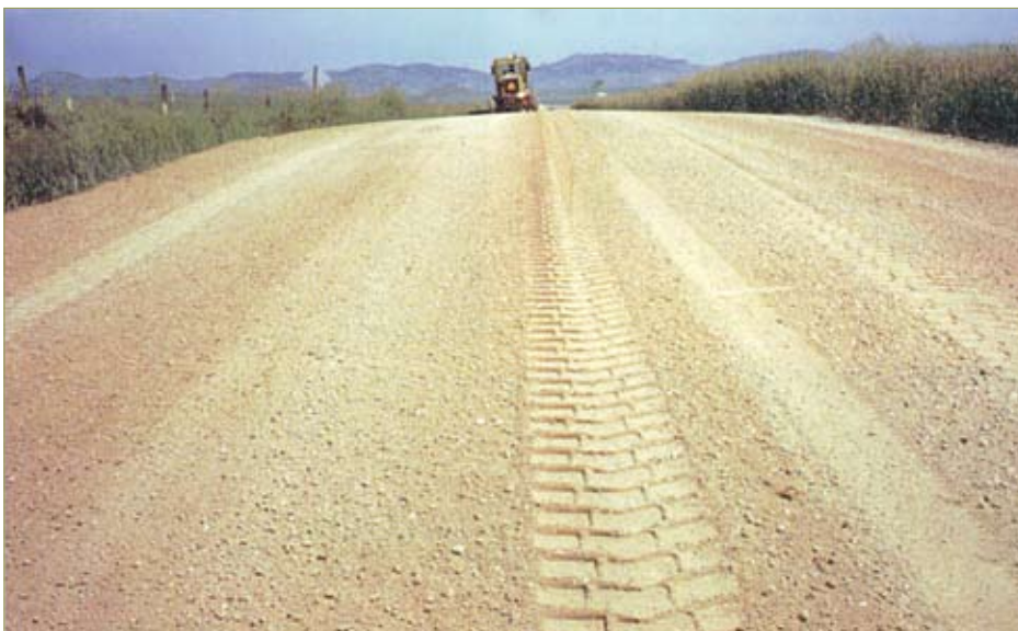
Figure 3–3. New granular surface (LTAP-SD)
