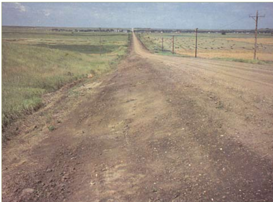
Figure 3–9. Foreslope height (LTAP-SD)
