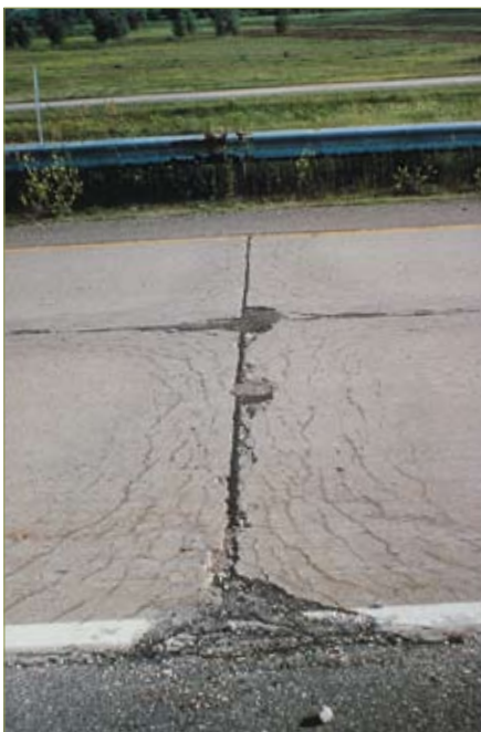
Figure 3-53. High-severity D cracks (FHWA)
