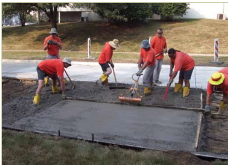
Figure 3-67. Vibratory screed (WDM)
