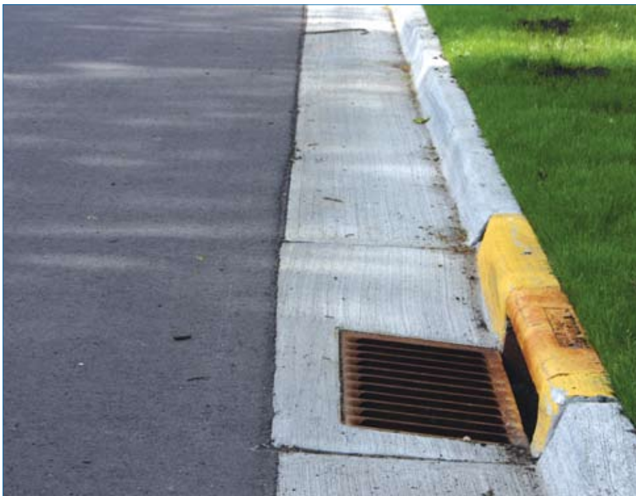
Figure 5-4. Water-tight joints at an inlet
