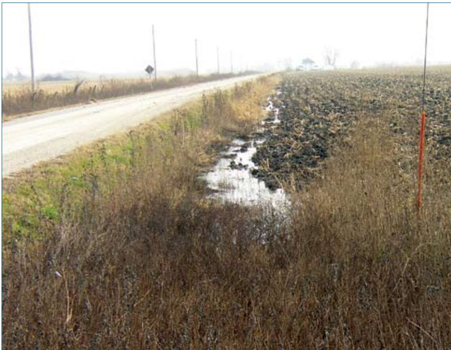
Figure 5–3. A flat ditch may not drain properly (Lee Co.)
