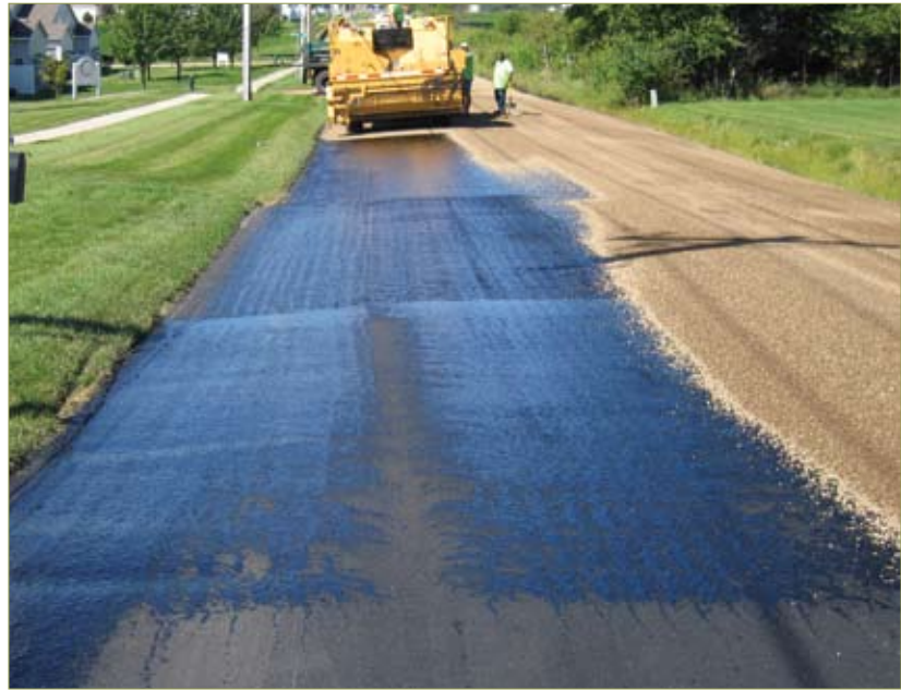
Figure 3–42. Asphalt binder and aggregate are used for seal coats (CCEE/ISU)
