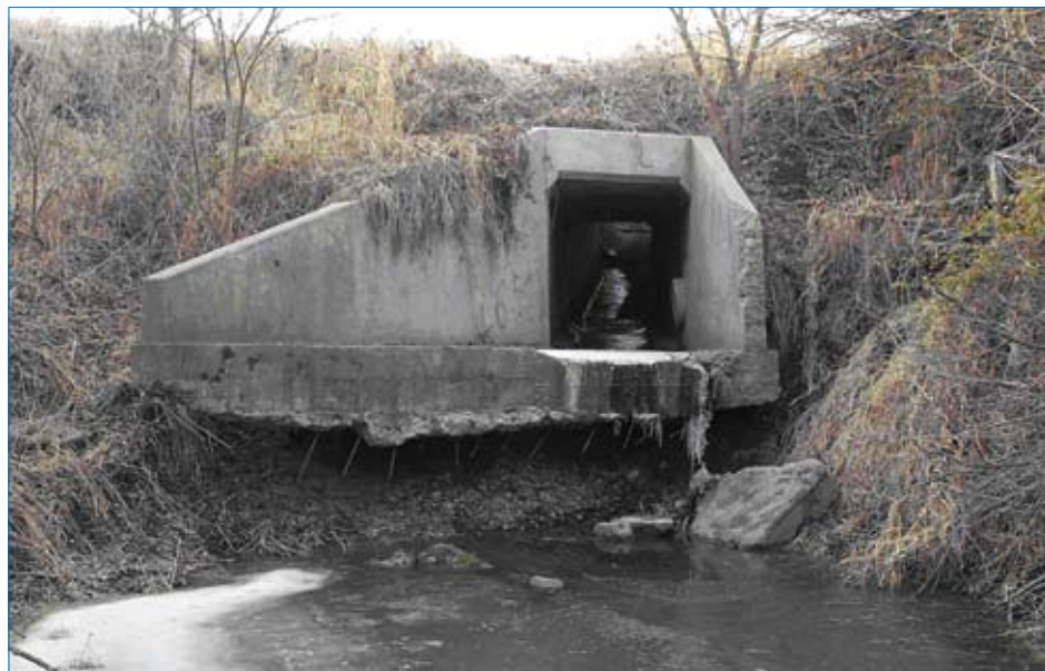
Figure 5–8. Deep scour at culvert outlet (Ettema, et al.)
