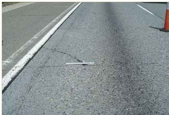
Figure 3–59. Corner break (FHWA)
