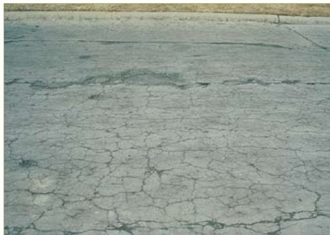
Figure 3-54. Map cracking (FHWA)
