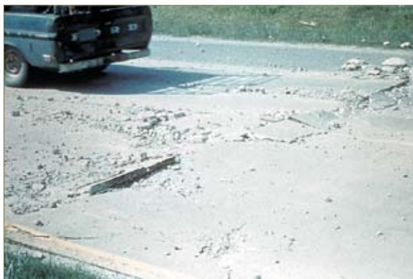
Figure 3–56. Blowup (FHWA)
