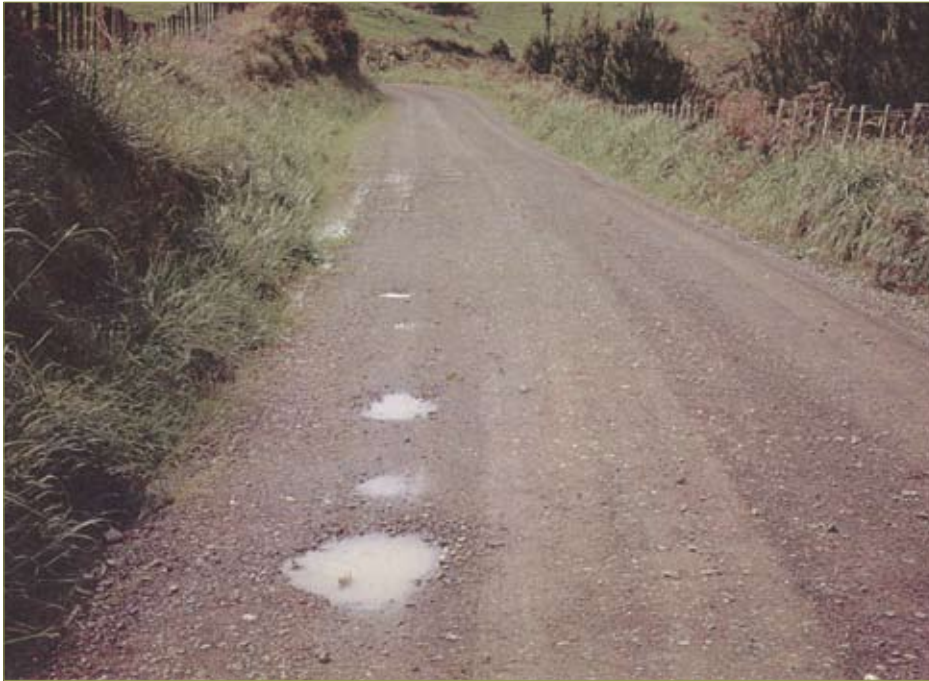
Figure 3–26. Potholes (LTAP-SD)
