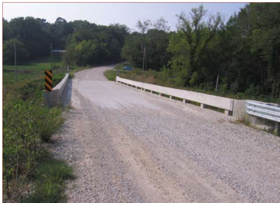
Figure 6–3. Gravel on bridge deck (CCEE/ISU)
