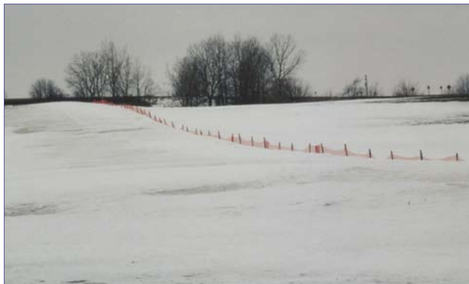
Figure 7–1. Properly installed snow fences cause snow to collect downwind (WDM)
