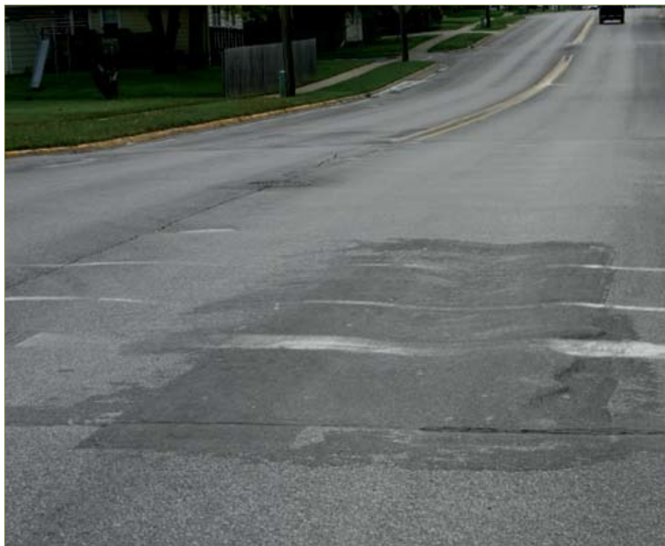
Figure 3–30. Rutting on an asphalt street
