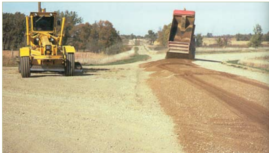
Figure 3-20. Placing new material on the roadway (LTAP-SD)
