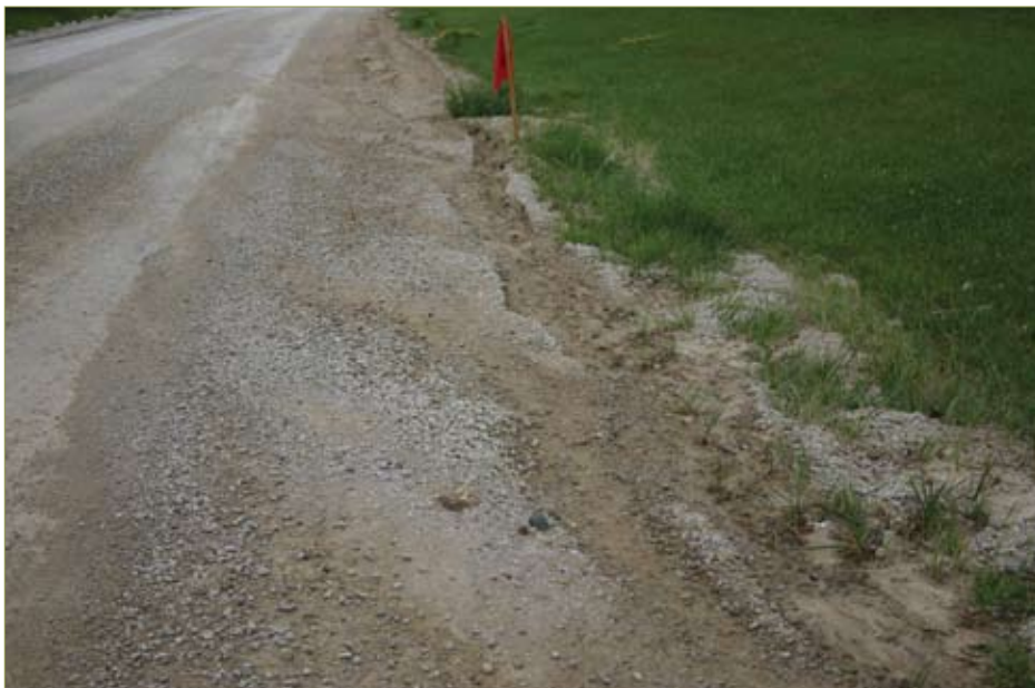
Figure 3-17. Windrow forming a secondary ditch
