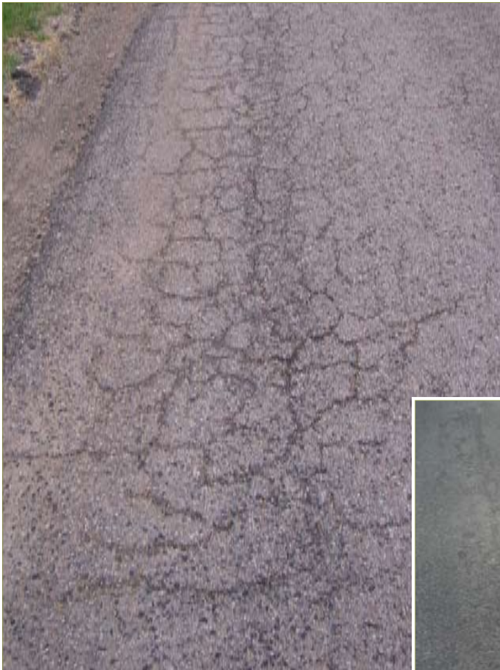
Figure 3–31. Fatigue cracking (CCEE/ISU)
