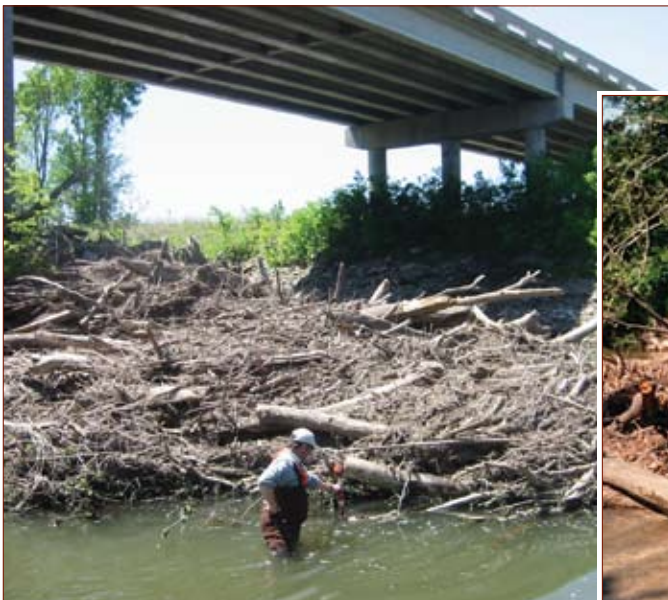
Figure 6-11. Debris collected around a pier (Ettema, et al.)
