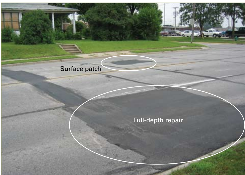
Figure 3–39. Surface patch and full-depth repair (CCEE/ISU)
