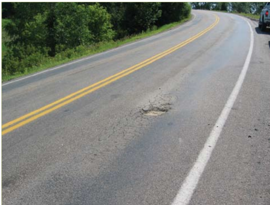
Figure 3–37. Pothole in asphalt pavement (CCEE/ISU)
