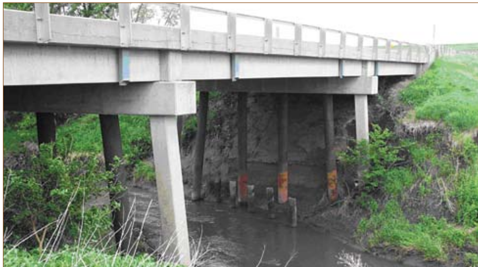
Figure 6–8. Erosion around base of piers (Ettema, et al.)
