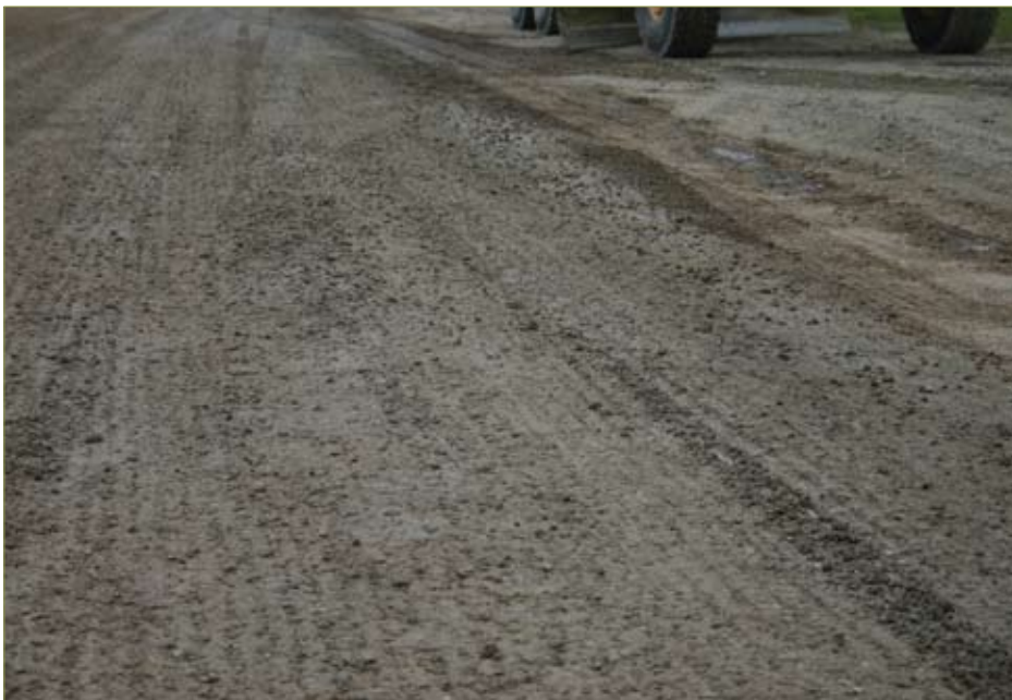
Figure 3–28. Adequate moisture for applying dust control material
