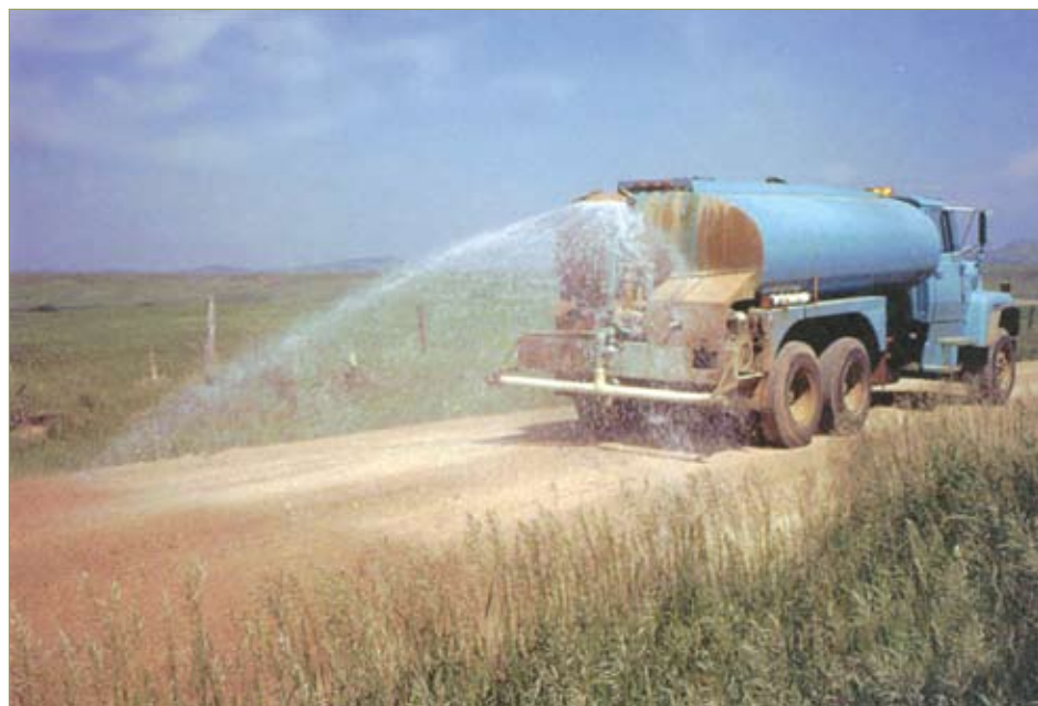
Figure 3-21. Adding water (optional) (LTAP-SD)
