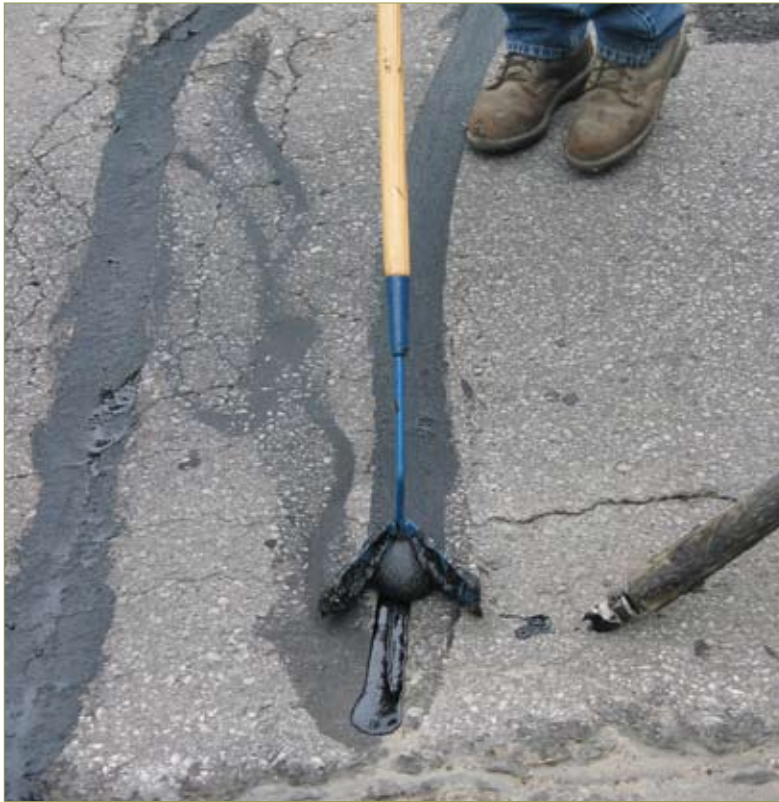
Figure 3–38. Crack sealing (CCEE/ISU)
