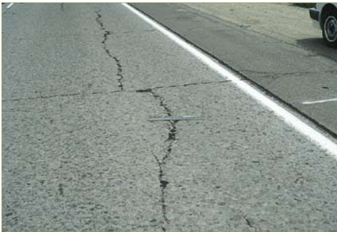
Figure 3-52. High-severity longitudinal cracks (FHWA)
