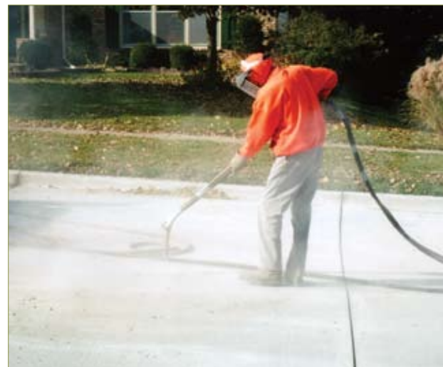
Figure 3-62. Cleaning joints before applying sealant (WDM)
