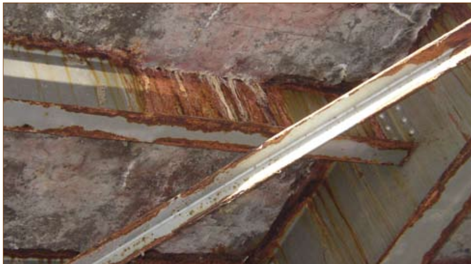
Figure 6–7. Evidence of deck seepage (Lee Co.)
