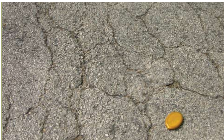
Figure 3–34. Alligator cracking (CCEE/ISU)
