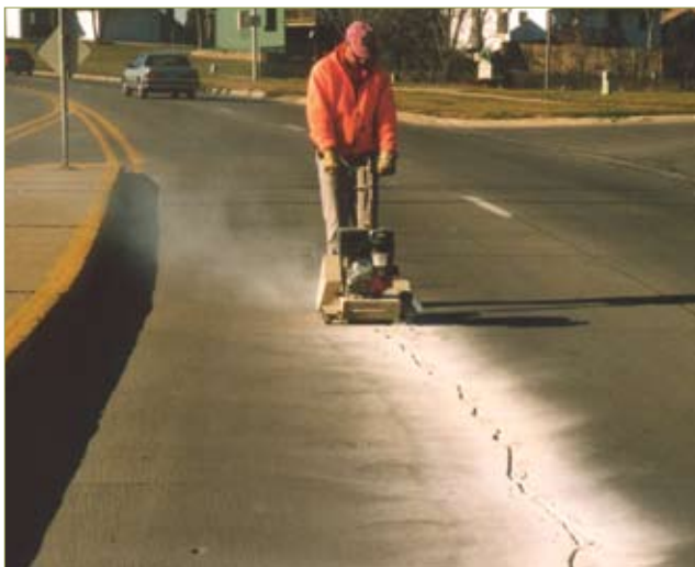
Figure 3-61. Routing cracks (WDM)
