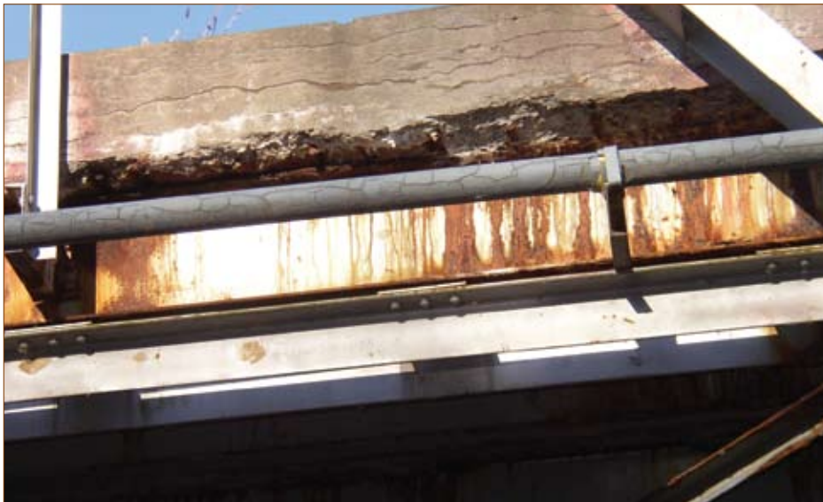
Figure 6–9. Corroded, discolored steel beams (Lee Co.)
