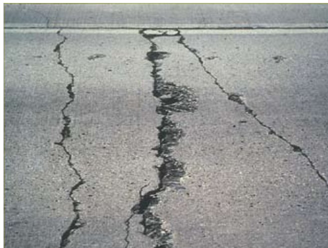
Figure 3–51. High-severity transverse cracks (FHWA)
