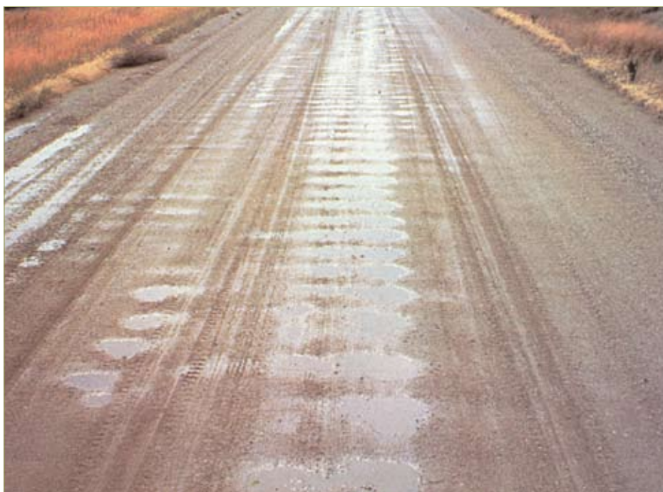
Figure 3–8. Poor crown shape (LTAP-SD)
