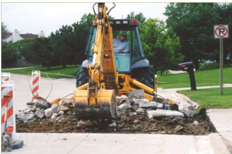
Figure 3-66. Removing full depth of slab (WDM)
