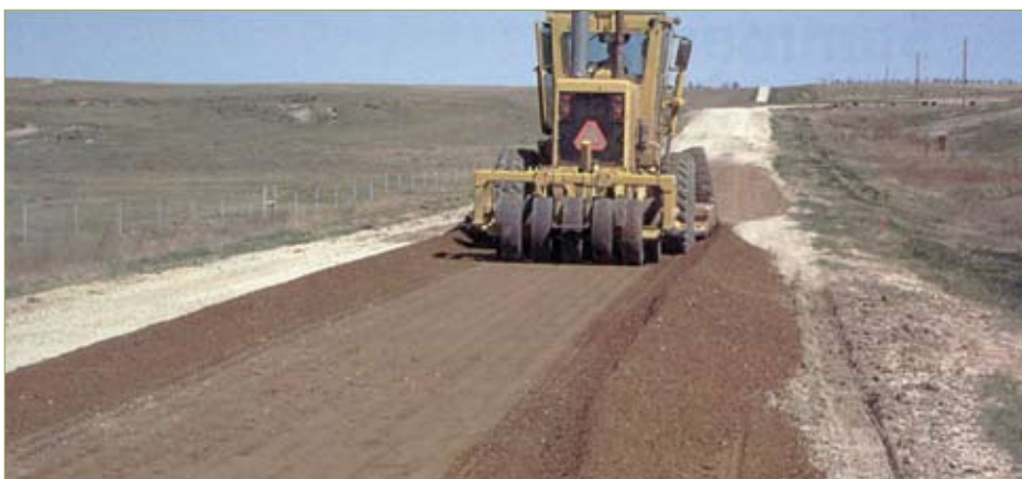
Figure 3–22. Compacting the new material (optional) (LTAP-SD)
