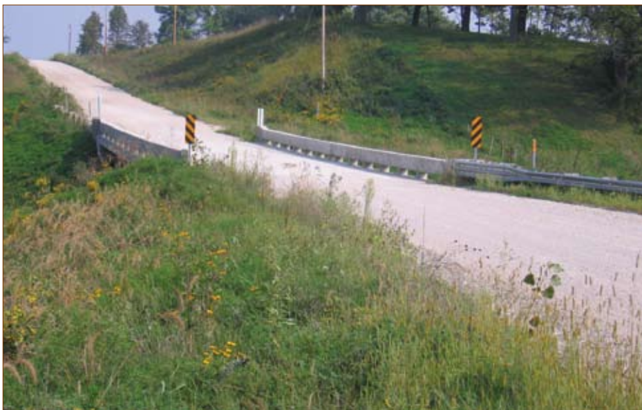
Figure 6–4. Visible object markers at a bridge (CCEE/ISU)
