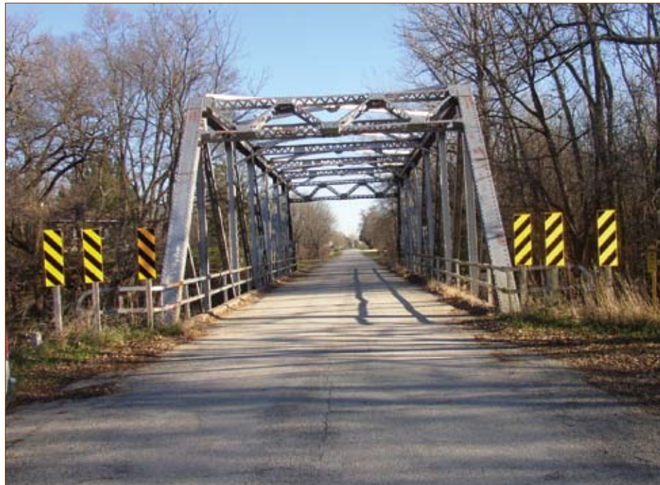
Figure 6–5. Well-aligned bridge trusses (Lee Co.)
