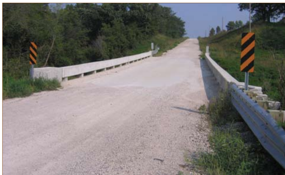
Figure 6–2. Overgrown vegetation at guardrail (CCEE/ISU)
