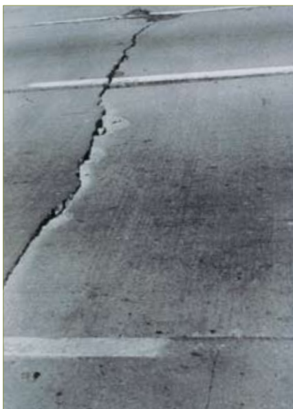
Figure 3–58. Faulting (FHWA)
