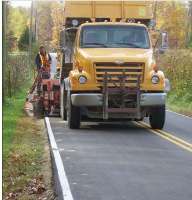
Figure 4–4. Repairing edge drop-off (LTAP-IN)
