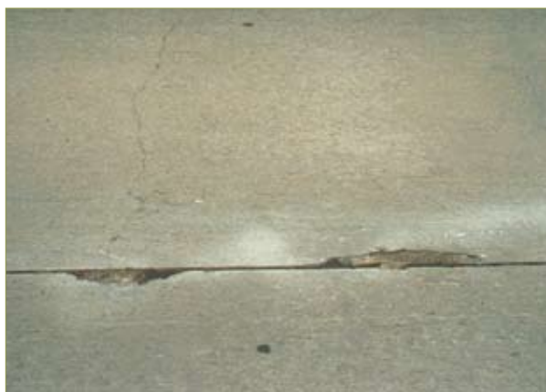
Figure 3–55. Spalling (FHWA)
