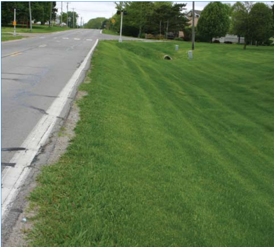
Figure 5-1. Ditch with good drainage
