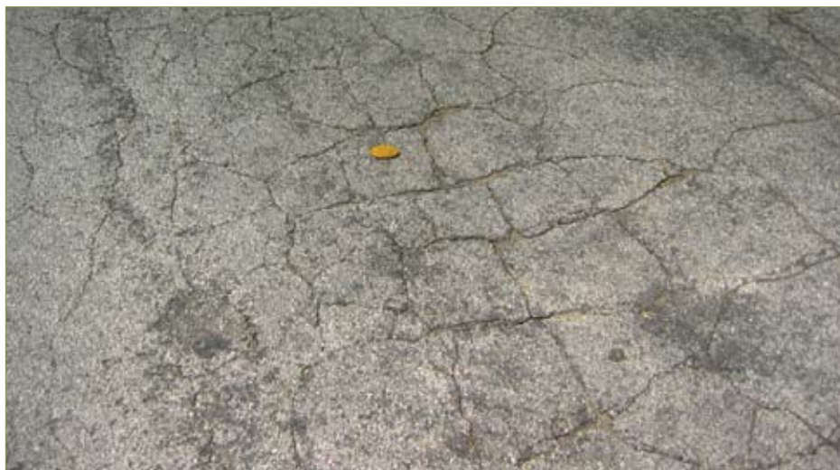
Figure 3–33. Block cracking (CCEE/ISU)
