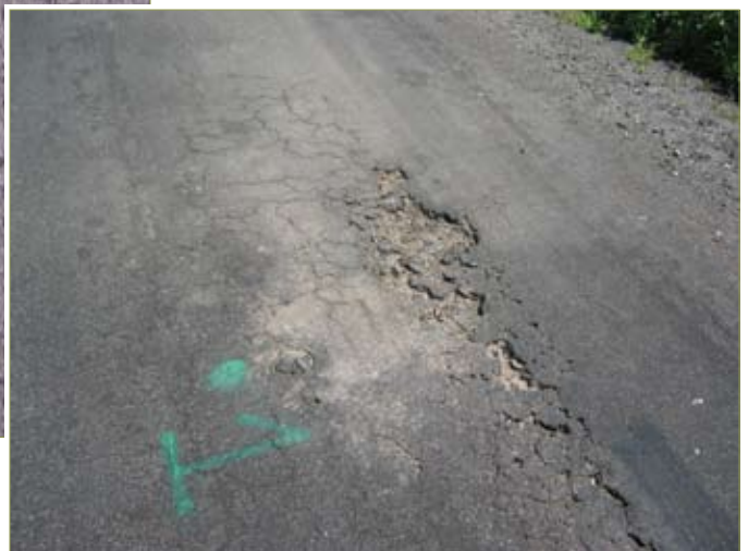
Figure 3–32. High-severity fatigue cracking (CCEE/ISU)
