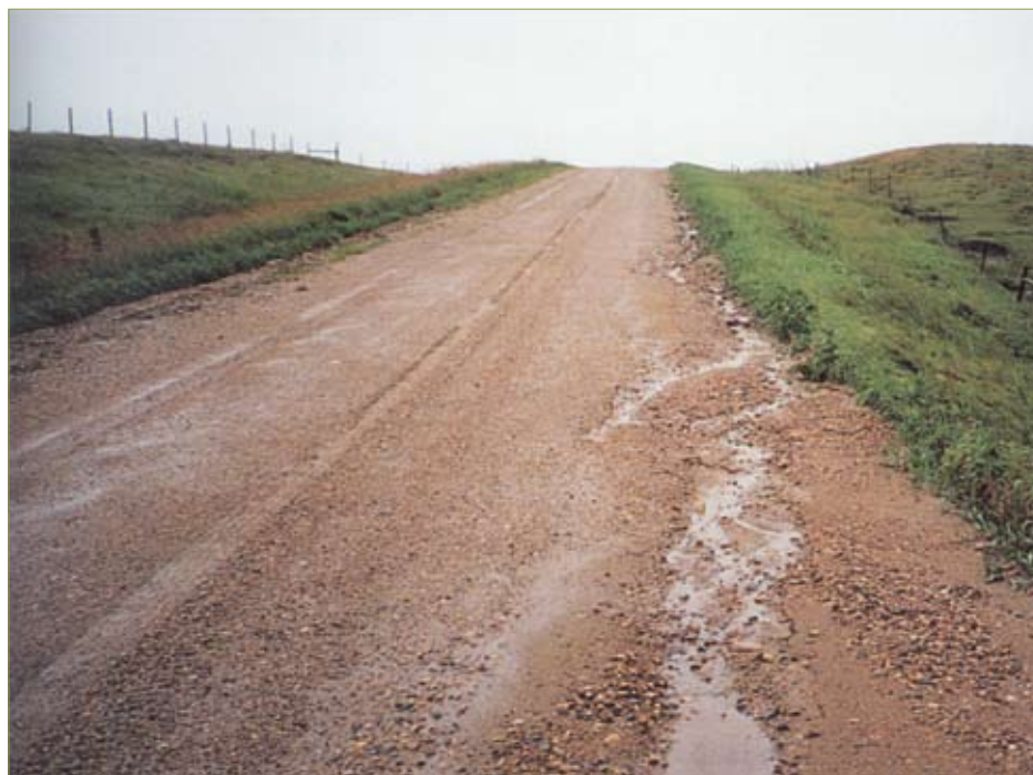
Figure 3–23. Secondary ditch (LTAP-SD)
