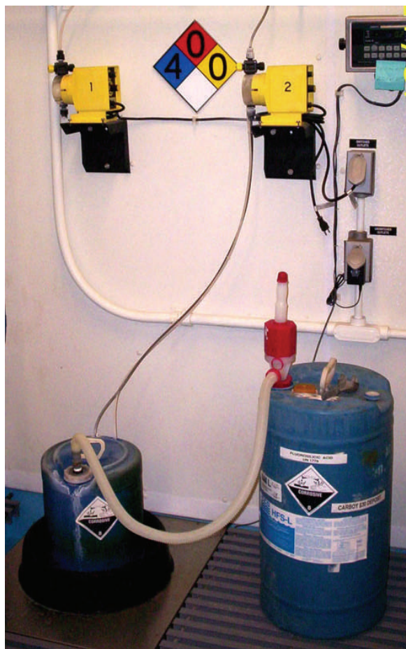
Water fluoridation devices, such as this one, add a therapeutic level of fluoride to community water supplies. In the case of high levels of naturally occurring fluoride, the amount of the mineral is reduced using osmosis.
