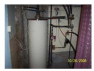
This is a picture of a water heater that the client had rigged to heat the building. The water heater used pipes under the floor to radiantly heat the house. The problem is that when they take a shower, all the hot water is expended and there is not hot water to heat the house.
