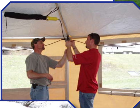
4. Electrical outlet strips and light fixtures are installed.
