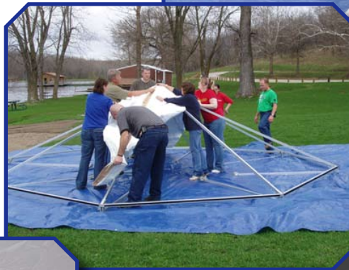
3. The roof (shown here) and sidewalls include an insulation package.
