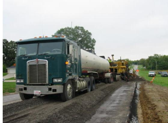
(b) Mixing process with foamed asphalt
