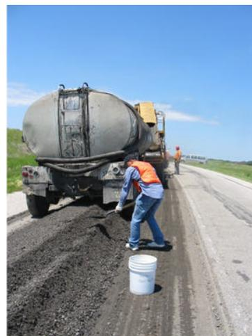
(b) Foamed asphalt mixtures
