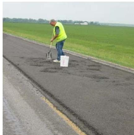
(b) Collection of foamed asphalt mixtures
