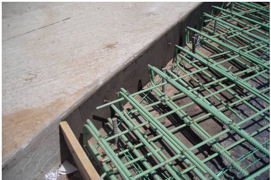
Installation of an improved bridge-to-pavement connection detail
