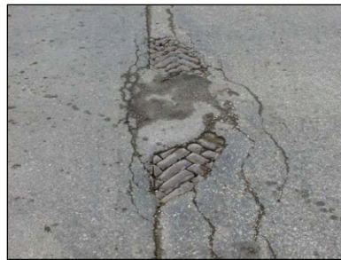
Asphalt Surface with Exposed Brick
