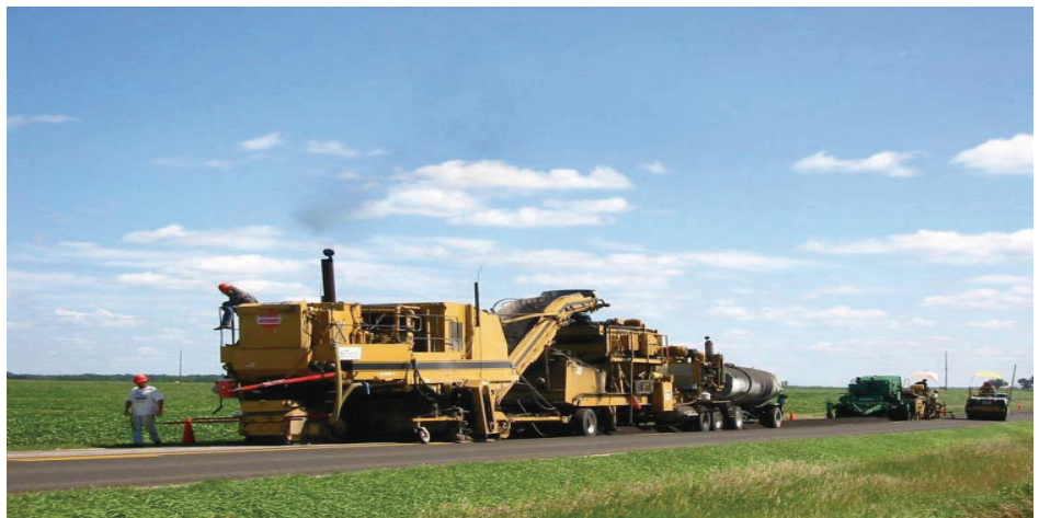
A typical CIR recycling train
