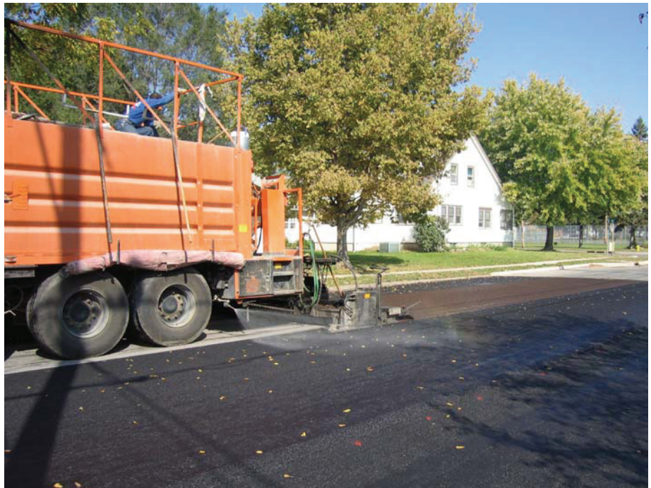
Micro-surfacing construction
