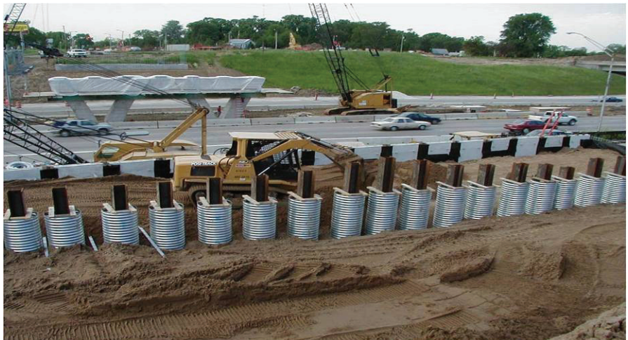
Abutment piles behind a MSE wall for a bridge over I-235 in Des Moines, IA
