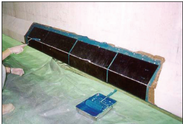
Installation of transverse CFRP jacket on Beam
