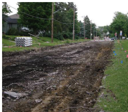
Existing non-uniform subgrade after pavement removal
